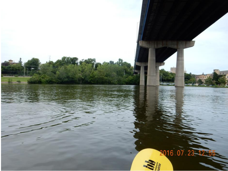
Photo 5 – looking back under Oneida Street Bridge
