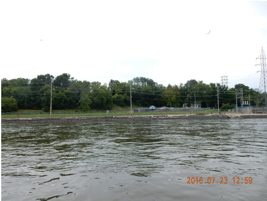
Photo 6 – looking towards the most-southwest point of the project boundary
