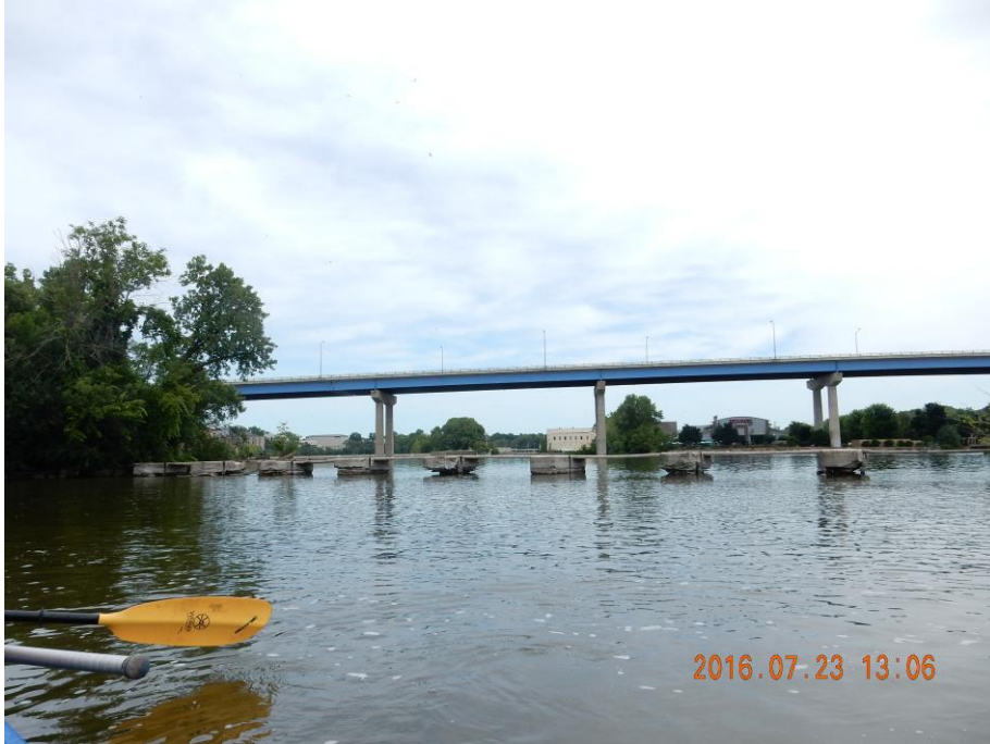
Photo 8 – looking at the upstream side of the train trestle
