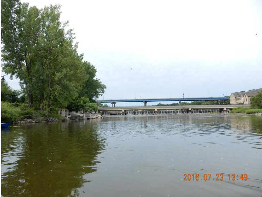
Photo 12 – looking upstream towards the Tainter gate structure
