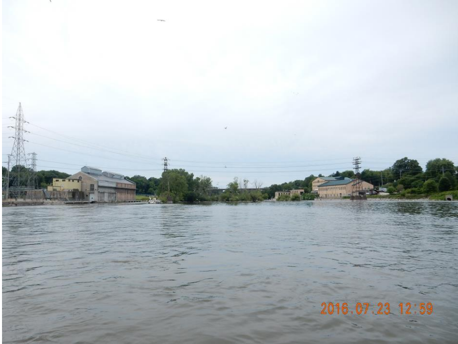
Photo 6 – upstream looking at upper dam
