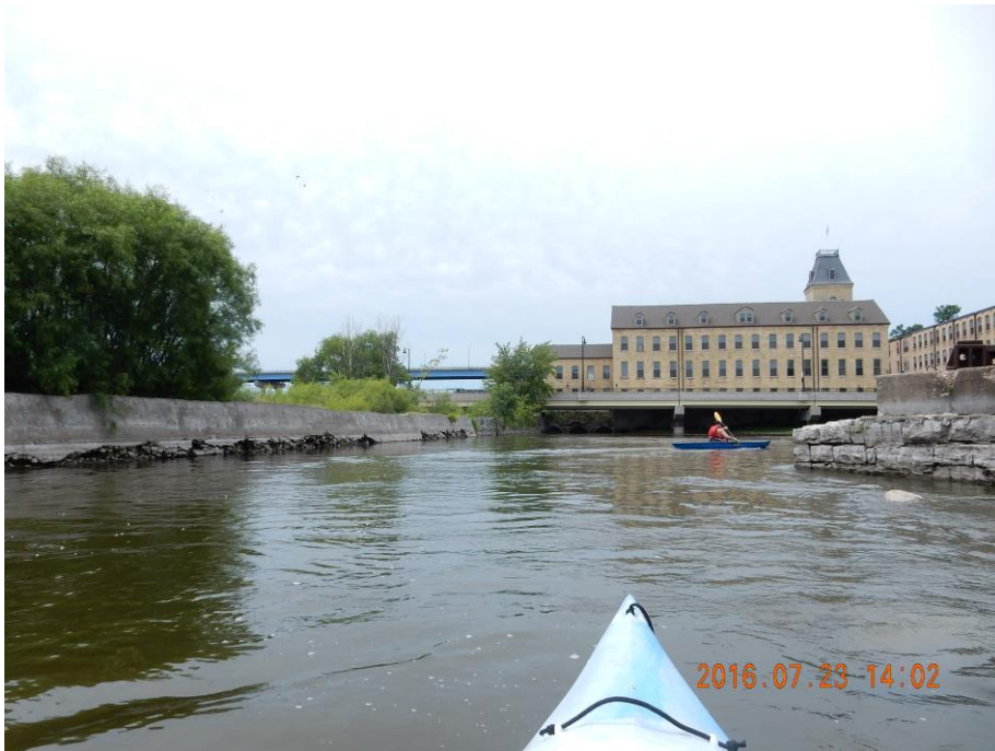
Photo 17 – looking upstream towards the old mill / powerhouse outflow
