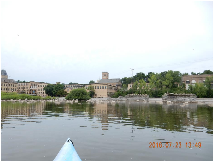
Photo 13 – looking north towards the island / training wall
