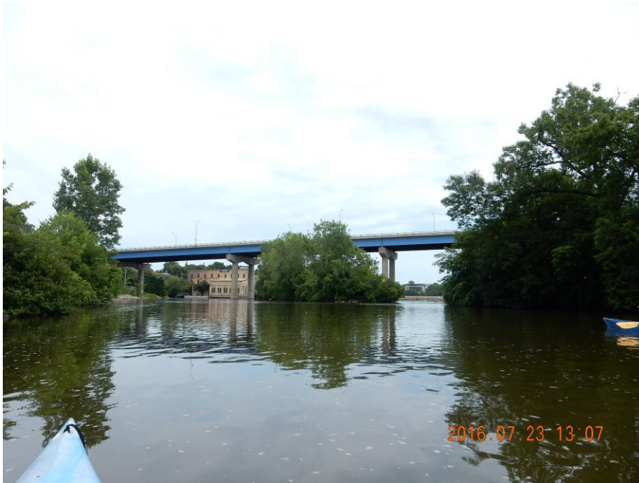
Photo 9 – looking downstream towards the north power canal Oneida Street Bridge
