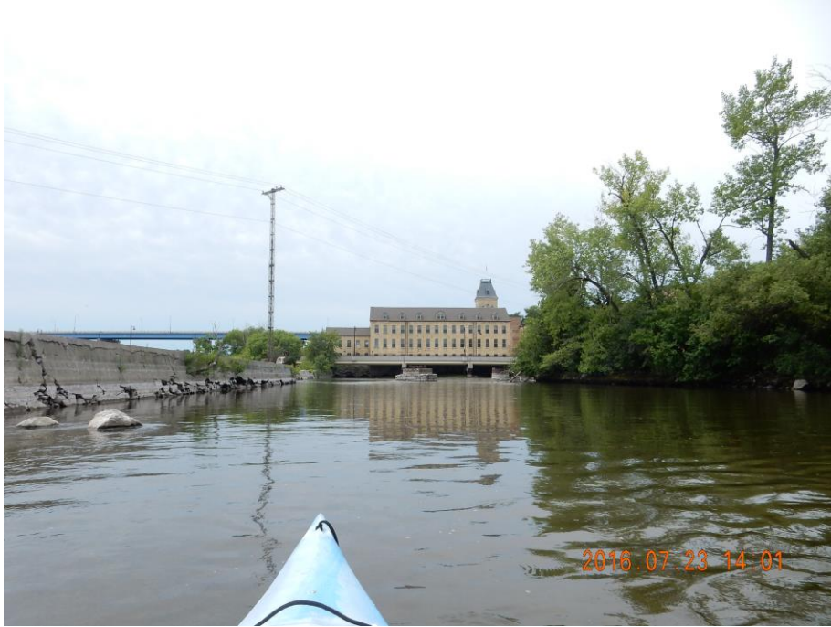
Photo 16 – looking upstream towards the old mill / powerhouse outflow
