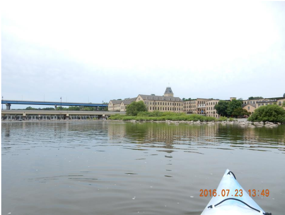
Photo 11 – looking upstream towards the Tainter gate structure and training wall
