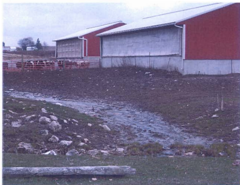
Figure 7 – NR 151 Violation Farm
