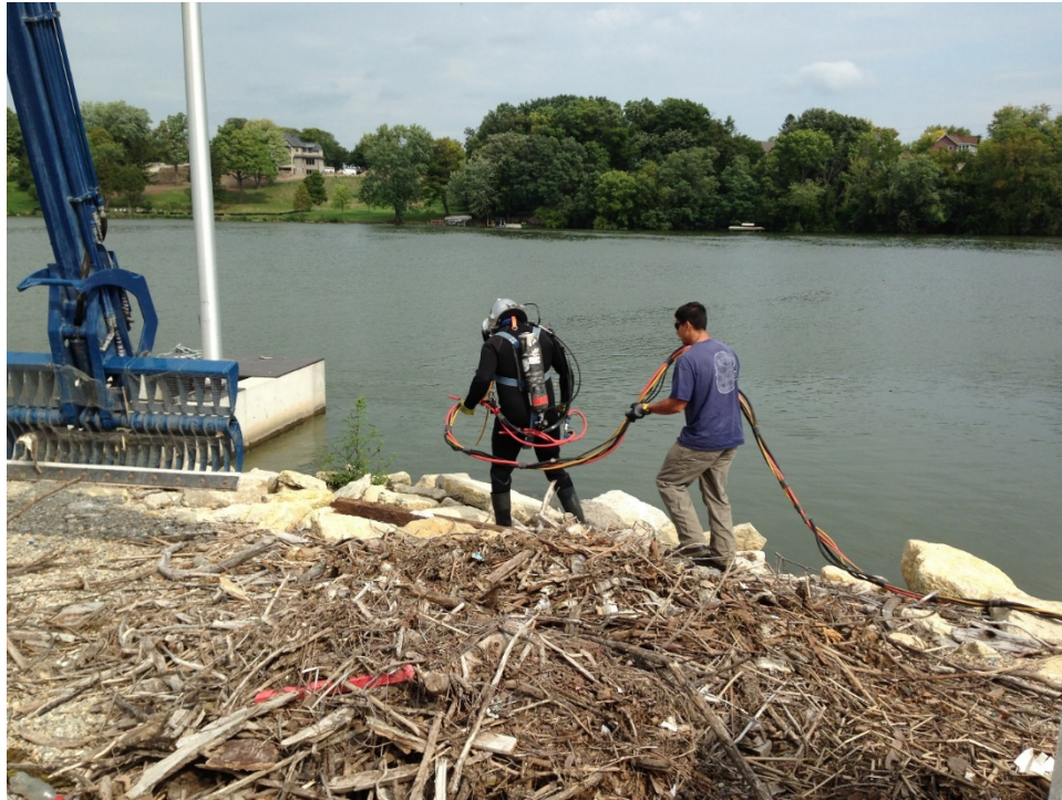
Photo No. 3 Diver preparing to retrieve detached Badger Upstream sonde on 9/16/16.
