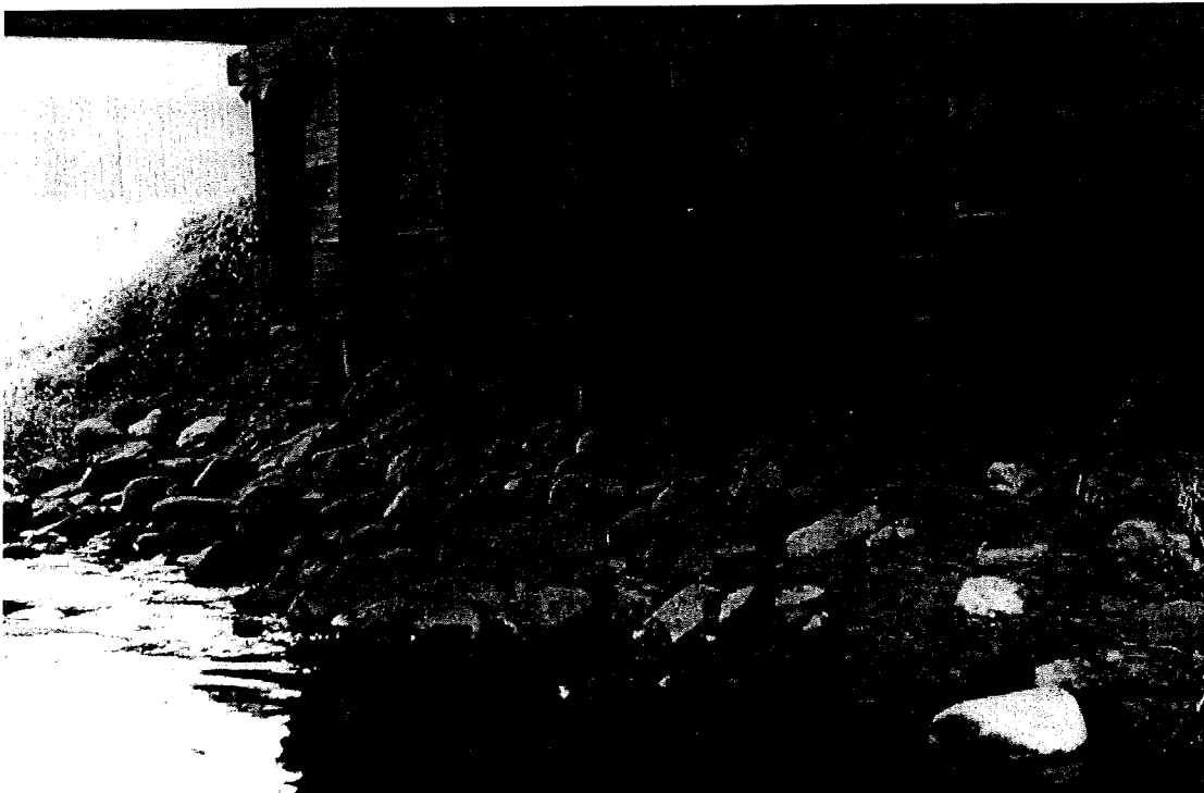
Photograph 8 : This Koshkonong Creek photograph was taken in April 1998 under the Highway T bridge. Rock riprap was placed here to protect the bridge footings from erosion. As much as 2 feet of sediment was measured over the riprap at this location.
