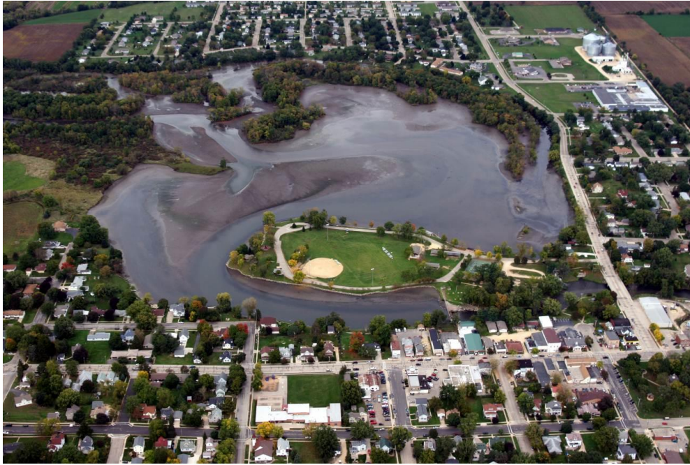
Photo 1: Lake Belle View Prior to Construction (2010 Drawdown)
