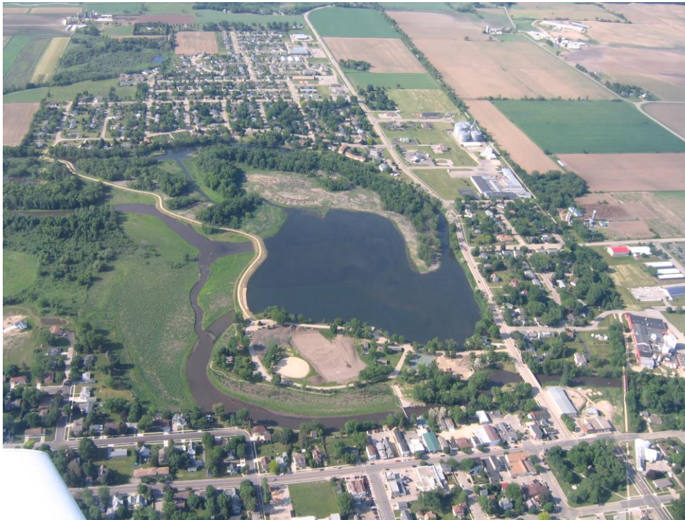
Photo 2: Lake Belle View After Construction of Separation Berm, Lake Deepening, and Habitat Earthwork (June 2011)
