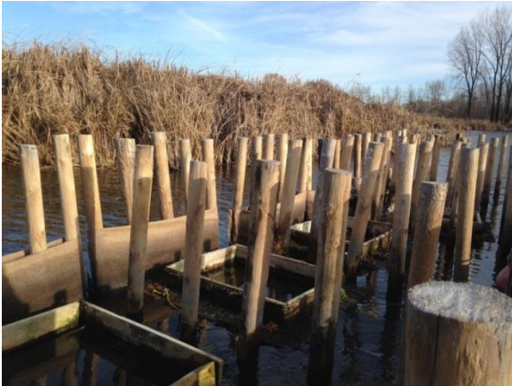
Wooden posts installed around planting boxes in fall of 2008 to prevent ice jam damage to the FBIs
