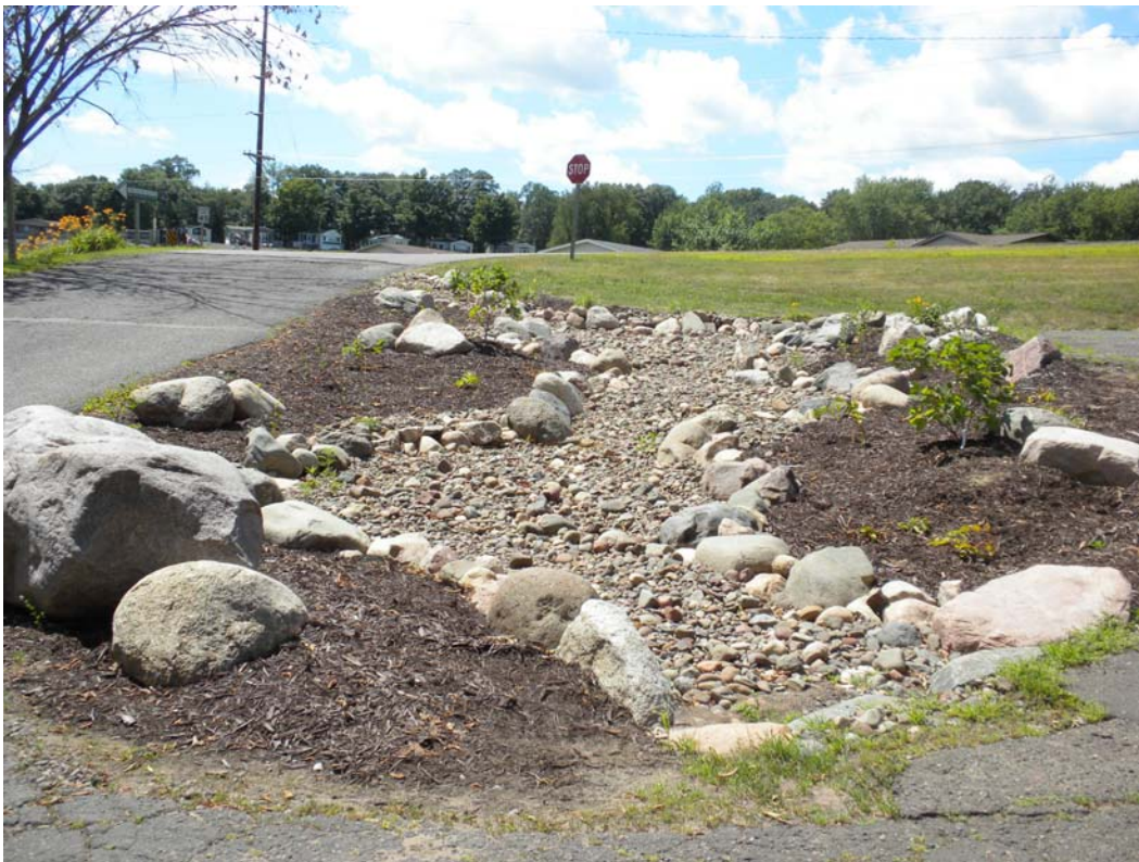
Balsam Lake Highway 46 Landing Rock Infiltration Pit. The diversion across the road was installed in 2013.
