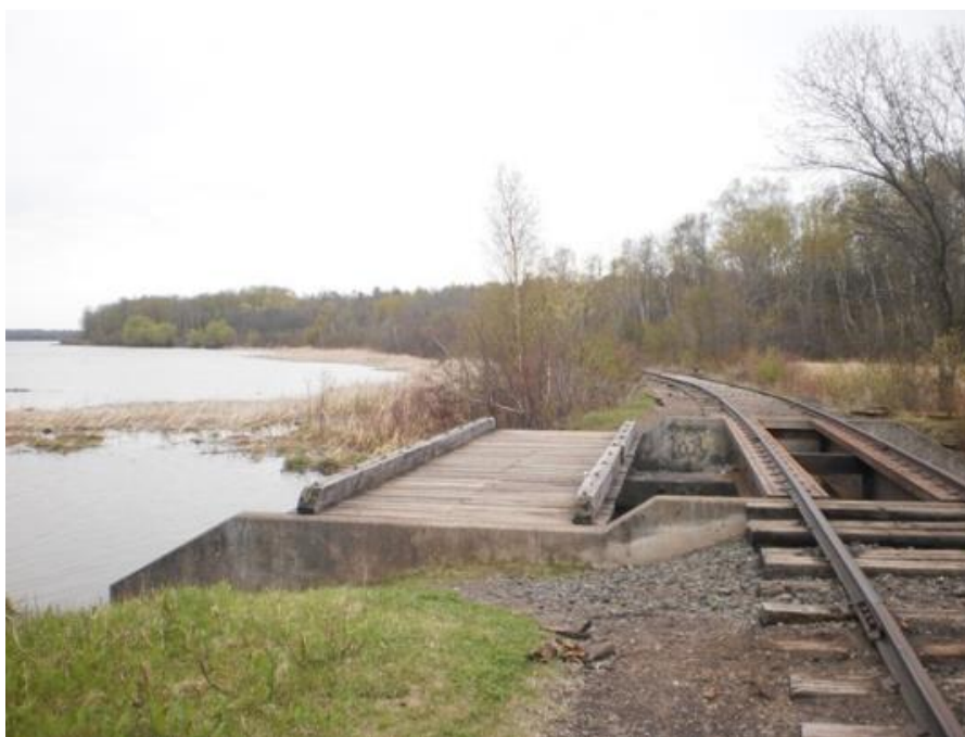
Figure 24. Railroad Bridge where Stewart Creek Enters the St. Louis River (CLYDE-ST).
