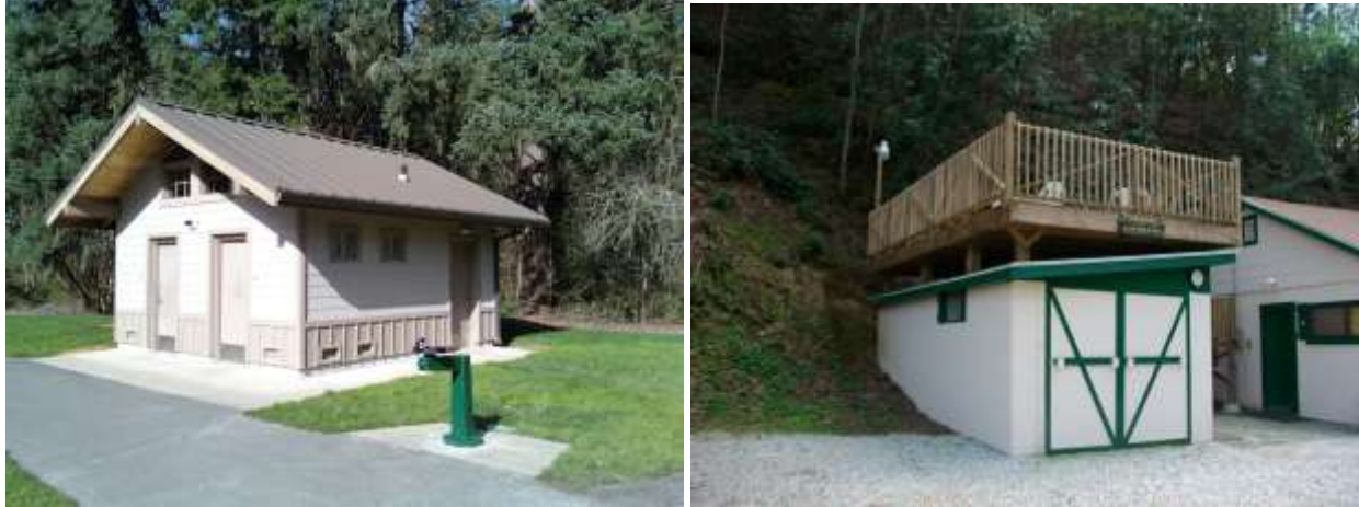
1 2 Figure 37 – Public Restroom – Hillsboro, Oregon (left); Observation desk on a small outbuilding (right) 3 (FontanaLakeNC.com)
