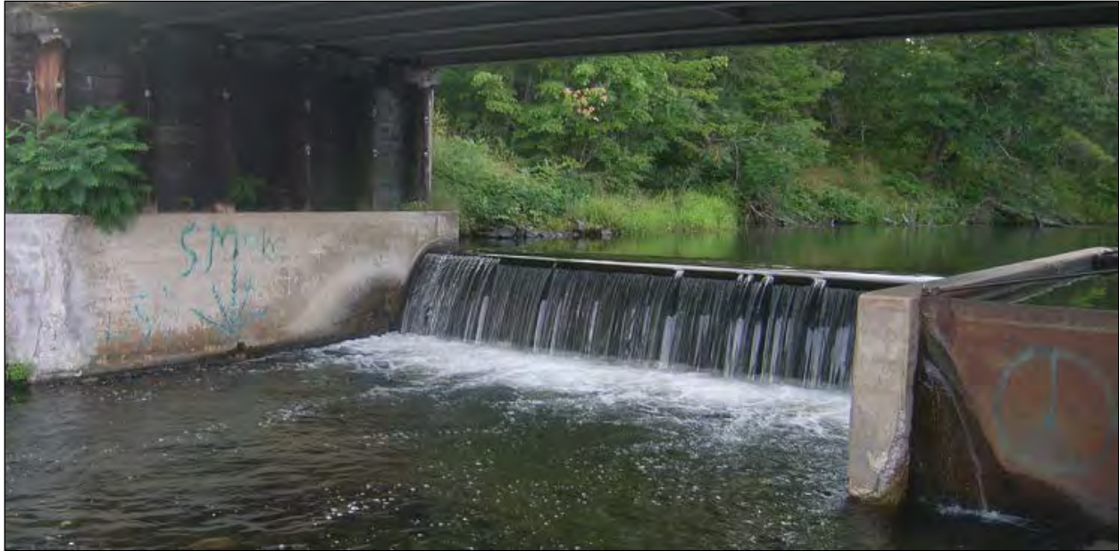
Figure 30 - Middle Eau Claire Lake Dam observed during August 2009. Observations were made during a period of substantial drought, and provide insight into low-flow conditions. Bridge above is for South Shore Road.
