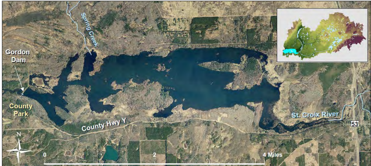
Figure 36 - St. Croix Flowage, formed by Gordon Dam, at the downstream extent of the SCHW. Aerial photo from 2009.
