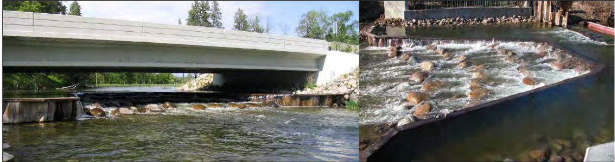
Figure 31 - Conceptual plan for fish passage at Middle Eau Claire Lake Dam via a rock rapids. This example project is located at Potato Lake near Park Rapids, MN (Source MnDNR 2010). A similar project could potentially be implemented at Middle Eau Claire Lake.
