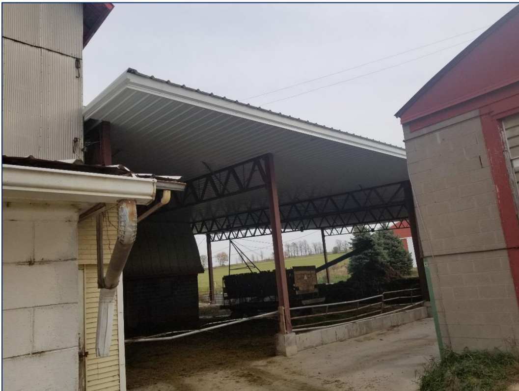
After: Constructed roof over feedlot and manure stack
