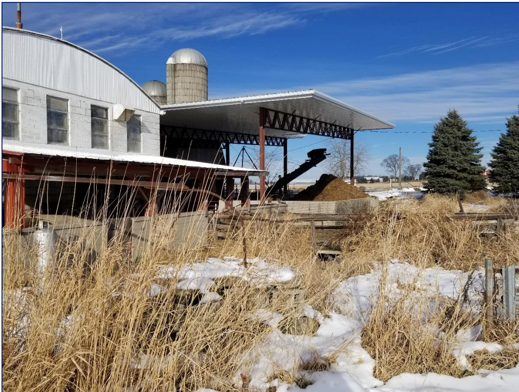
After: Covered Feedlot and stacking area
