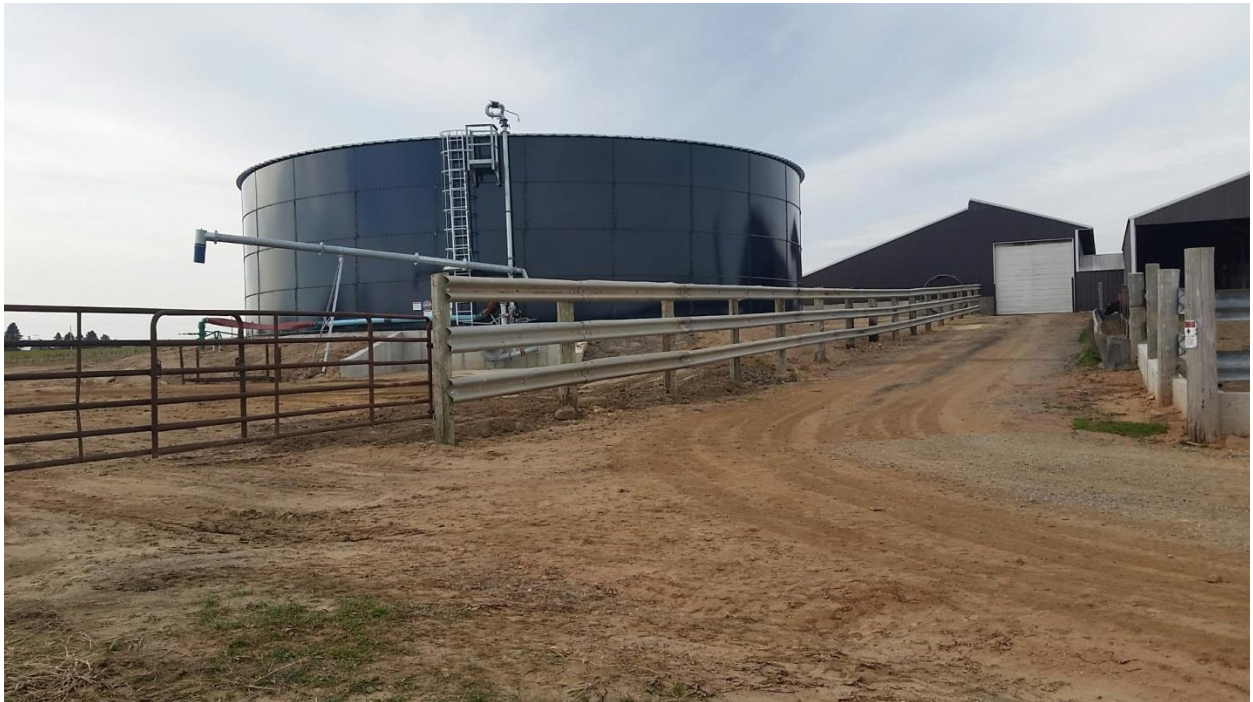
Figure 8: Completed Slurrystore manure storage structure where manure lot runoff and "hot" feed leachate is pumped into automatically (after in Nov. 2016)
