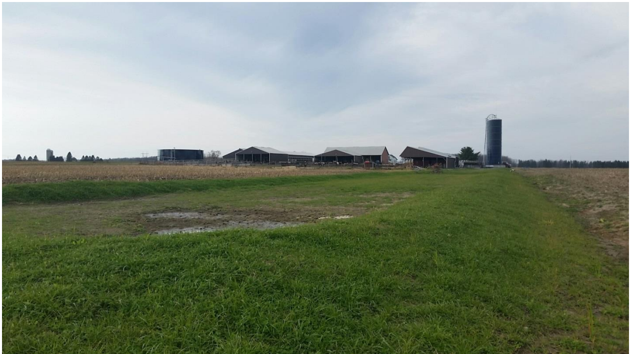
Figure 6: Mostly established 3-cell VTA and completed Slurrystore manure storage structure in middle left background (after in Nov. 2016)
