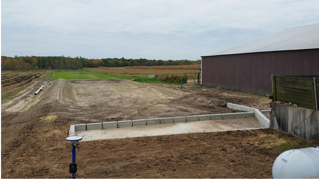
Figure 5: 3-cell VTA designed to contain 24-hour 25 year storm event after "hot" leachate is pumped into new manure storage tank (after in Oct. 2016)
