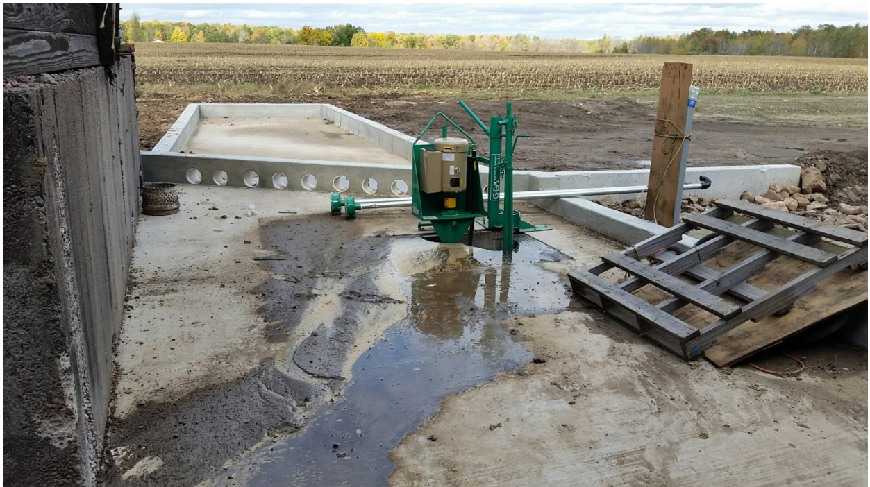
Figure 4: Feed leachate runoff flowing into PLC pumped tank designed to catch "hot" leachate and allow rain diluted runoff onto VTA (after in Oct. 2016)
