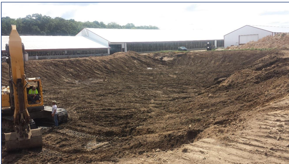
All waste removed from existing storage facility
