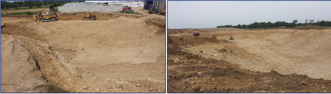
Grading and shaping earth for new concrete lined storage facility
