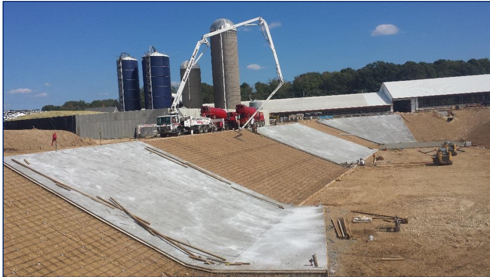
Pouring the many sections of a new lined facility
