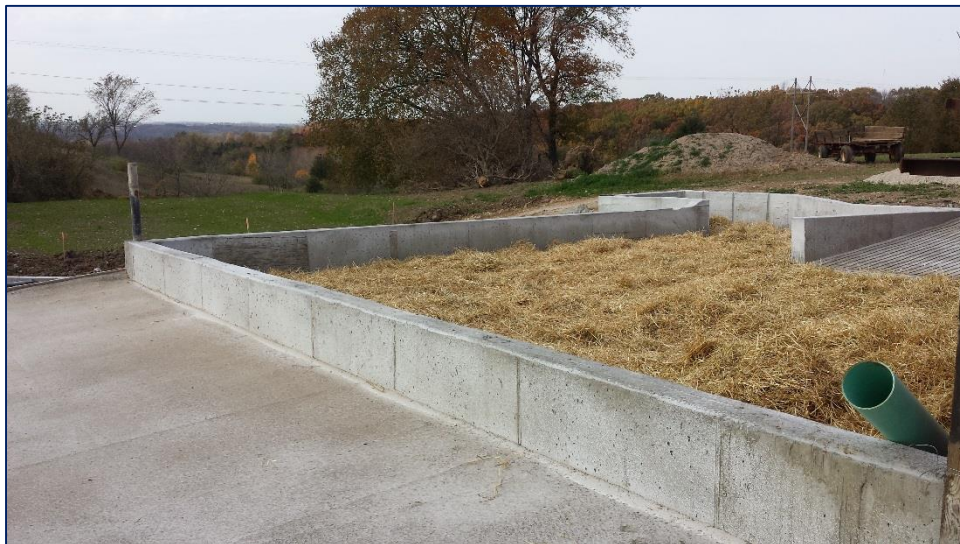
Constructed settling basin (straw in picture to protect concrete from freezing)
