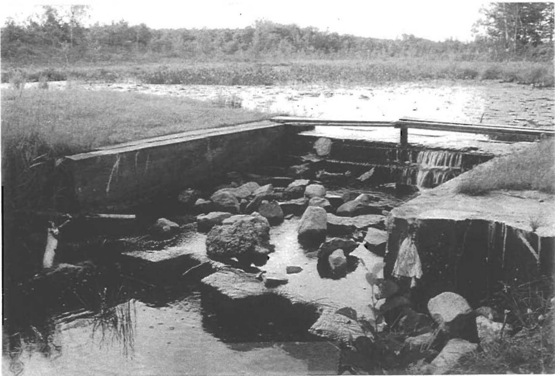
Figure 6. The Crooked Lake Dam. Accessible from Tar Dam Road.
