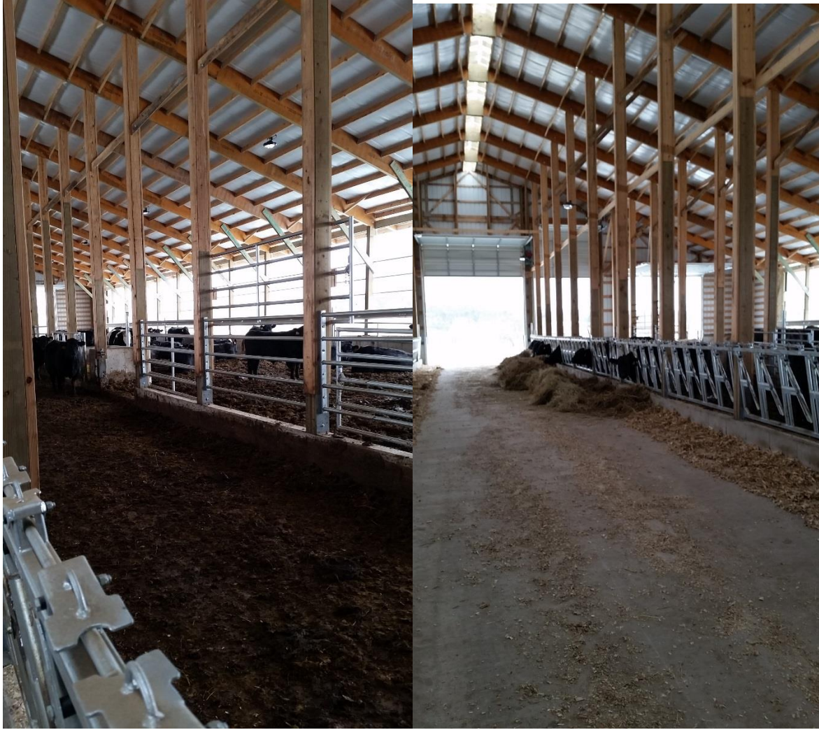
Roofed Barnyard in use – 12/2017
