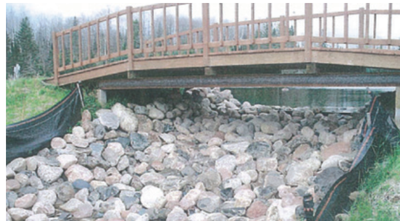
Above: This is a typical rip-rap rock chute dam for a high head. The steel sheet pile can be seen under the bridge. This dam will look very natural and in keeping with our environment. Low maintenance bodes well in considering the longevity of this dam. Construction costs are low while maintaining a high quality structure.
