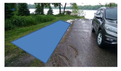
Install rock infiltration area under parking areas. Keep shallow to maintain separation to water table (approx. 8ft  $\times$  40ft.  $\times$  0.5 ft = 160 ft<sup>3</sup>) **6 yards**
