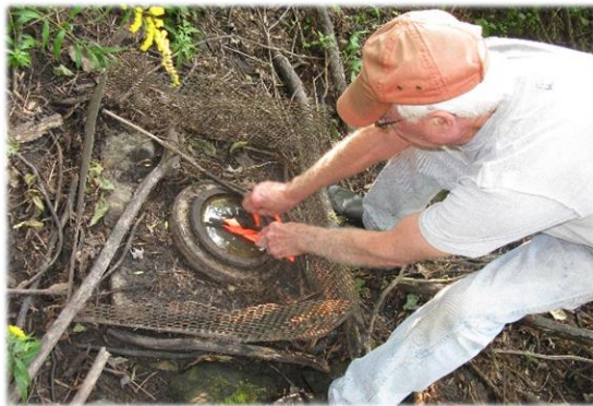
Existing connection between Fish Creek and the smaller pond.
