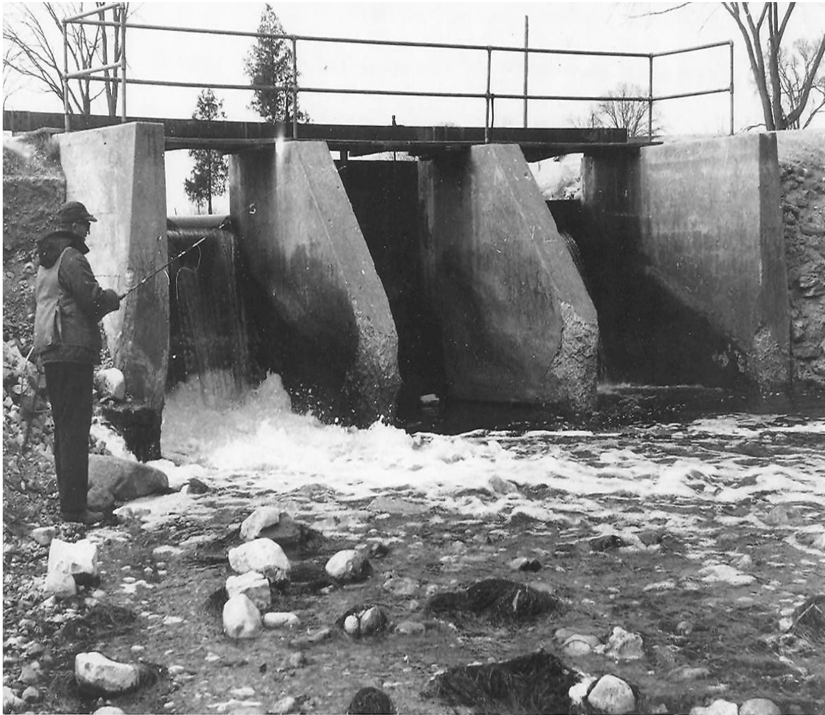
Figure 1-3. Forestville Dam in 1934
