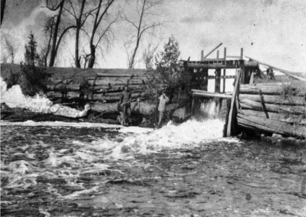
Figure 1-2. Forestville Dam in 1918
