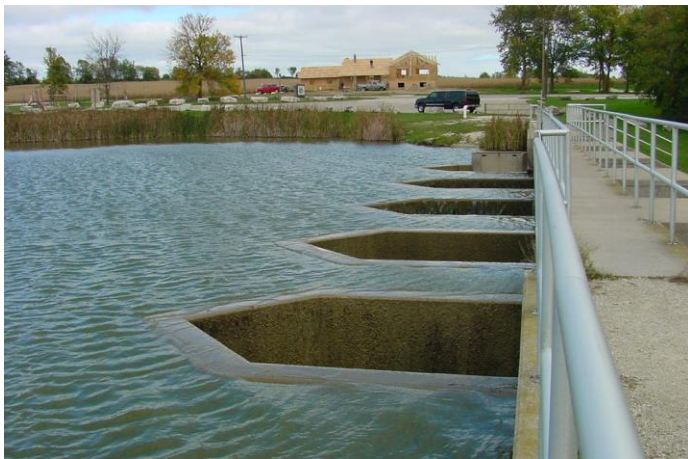
Figure 1-5. Dam Overflow Spillways
