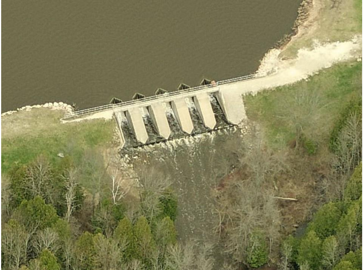
Figure 1-4. Forestville Dam in 2011
