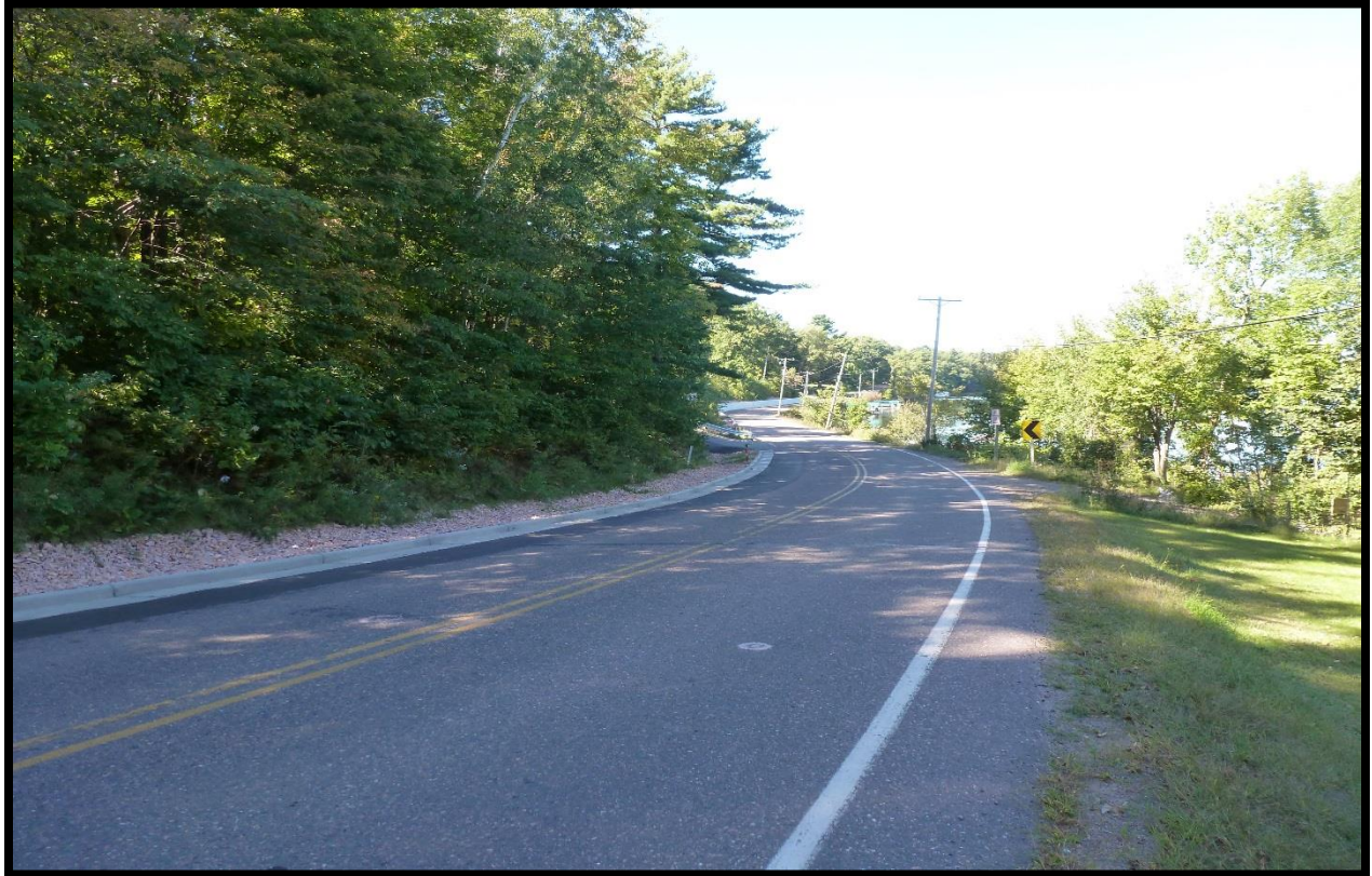
AFTER Looking north
