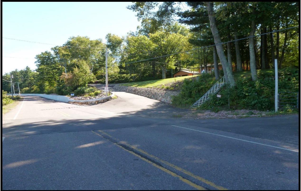
AFTER Looking southeast
