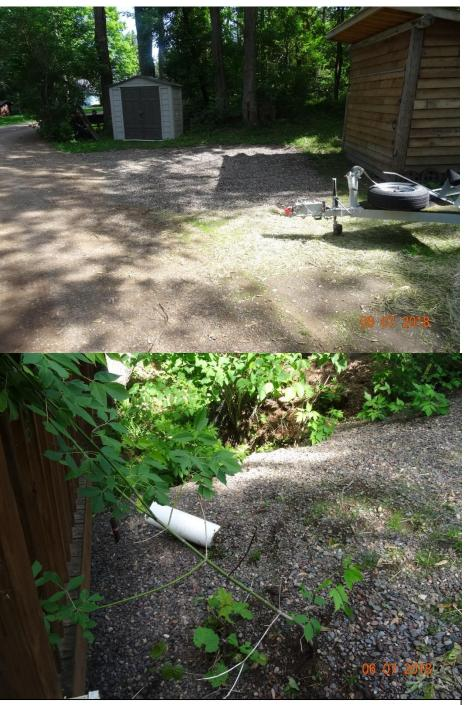
AFTER: Runoff flows to rock infiltration pit with PVC overflow. Capacity of pit and infiltration to substrate allows little discharge to the channel to Bone Lake.
