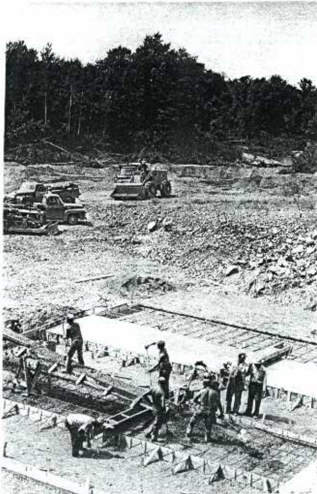
Work begins on Mead Dam-1954 Picture courtesy Hoffman Family
