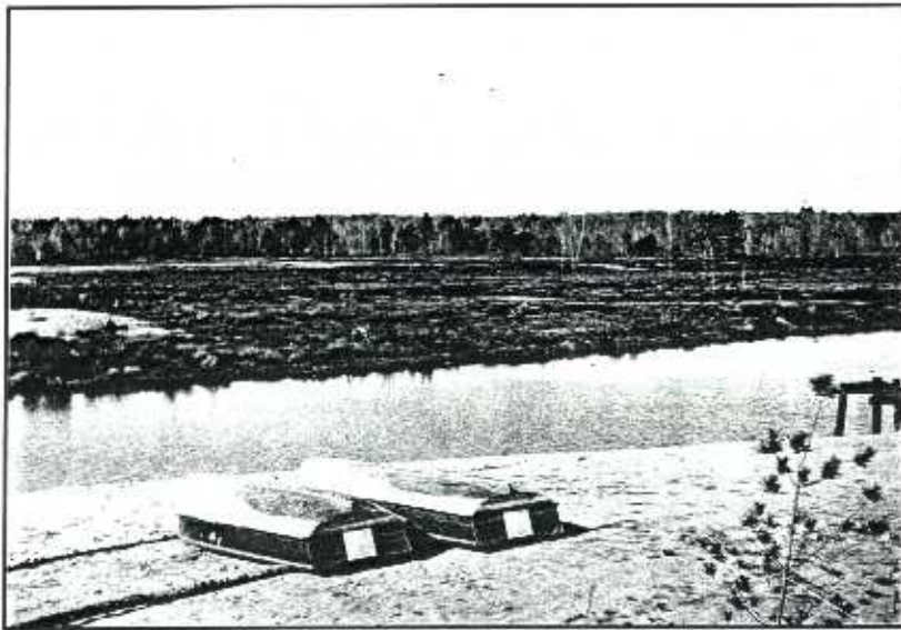
Lake drained for dam work in front of Hoffman's (next to dam)
