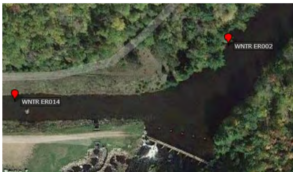
Figure 24. Impoundment erosion site 2017.
