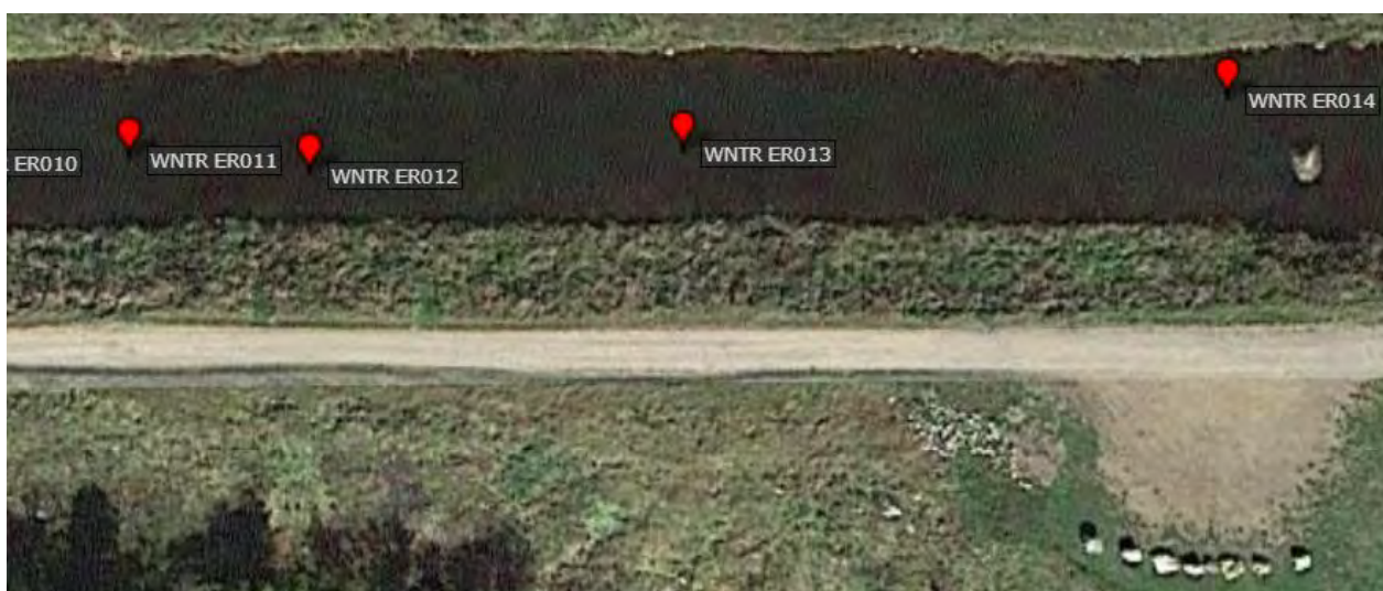
Figure 23. Bypass reach erosion sites 2017.
