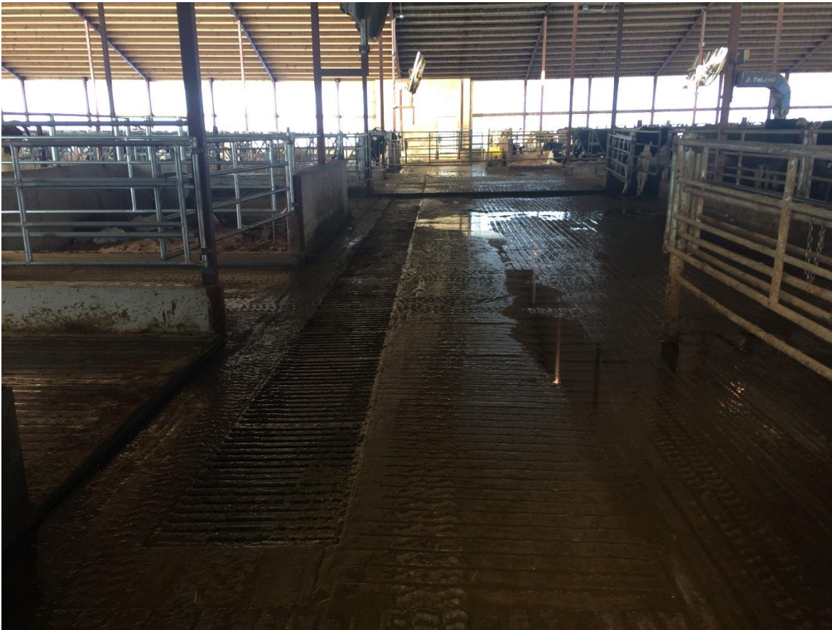
Waste Transfer – 18" Auger Channel with sand auger & slatted grating
