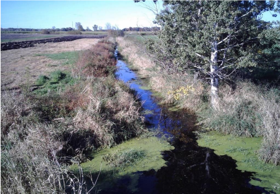
Photo 2: Thiel Creek at County N facing upstream. Photo taken by D. Bolha on October 11 th , 2017.
