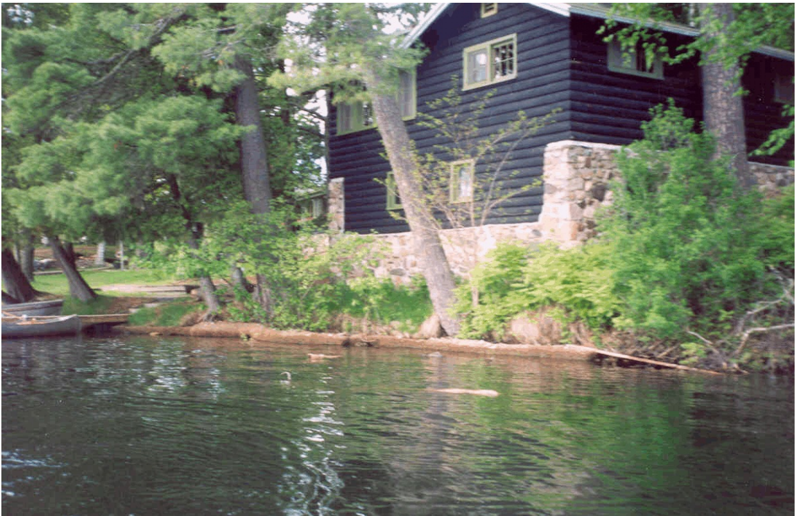
Shoreland erosion control effort using bio-logs on another lake in northern Wisconsin in 2004.
