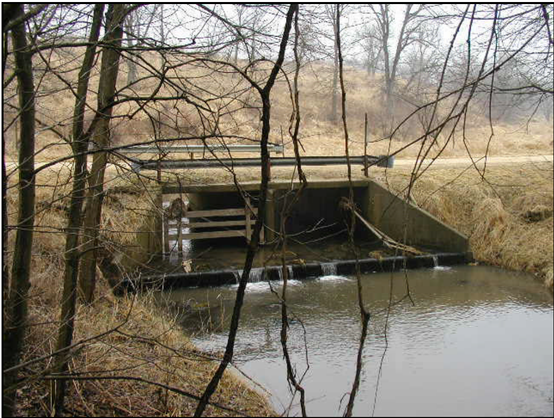
Figure A-8. Oversized bridge culvert on Snowden Branch near Station 2
