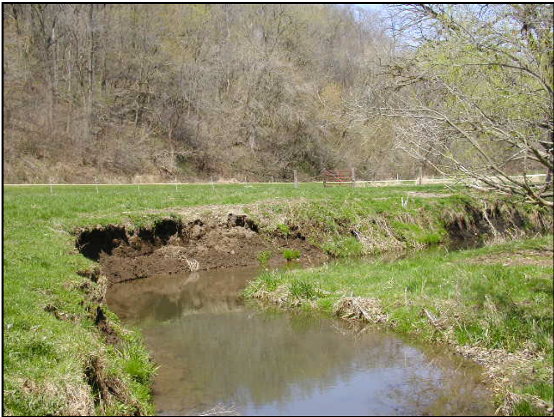
Figure A-6. Typical bank erosion in Snowden Branch (approximately 1m high)
