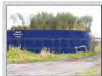
Abandoned waste storage structure.
