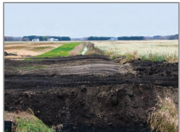
Figure 12. Finished Ditch Plug with Crown in Middle
