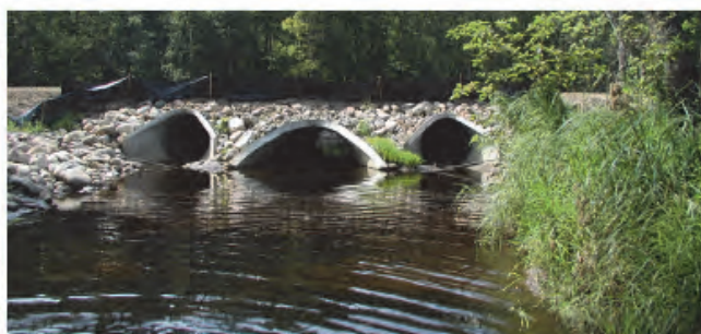
Properly sized and placed culverts.
