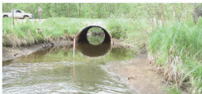
Undersized culvert.
