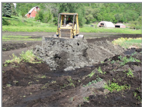
Figure 2. Shallow Ditch Being Filled
