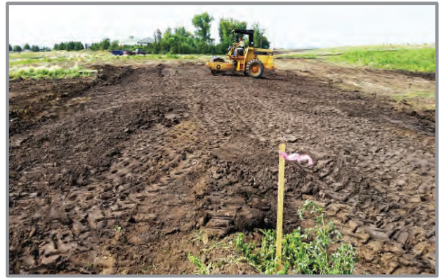
Figure 11. Compaction of Constructed Ditch Plug
