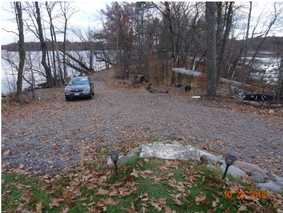
grading and rock diverted runoff to the infiltration pit
