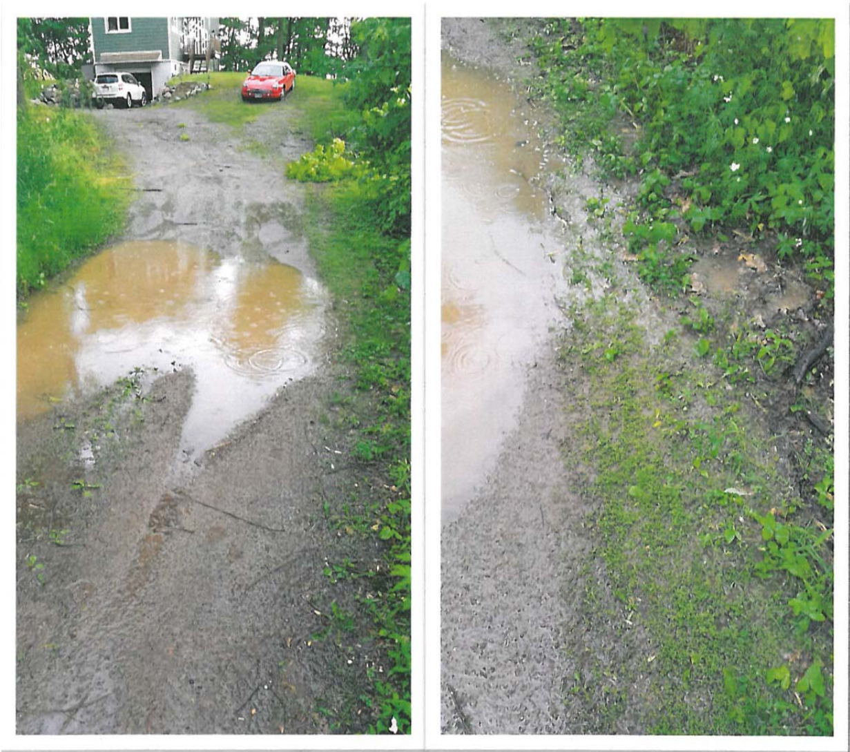
Picture 1: View south from low area
