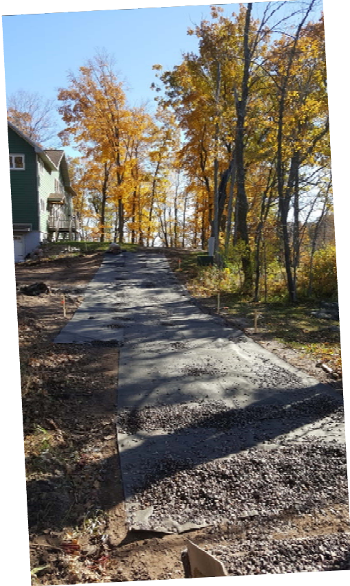
grading and rock diverted runoff to the infiltration pit
