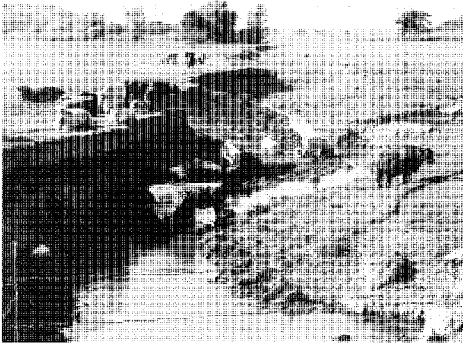
Streambank erosion from grazing
