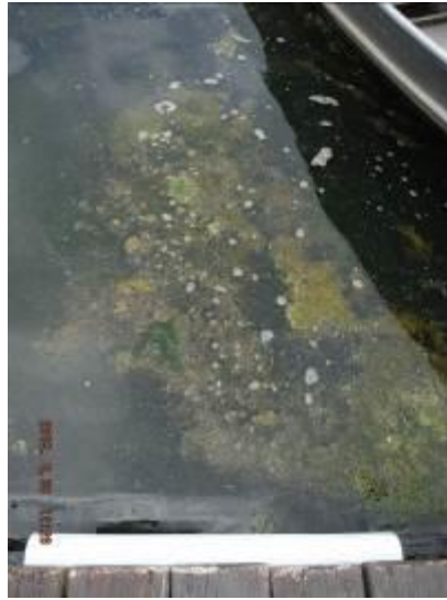
Concession dock – N side
