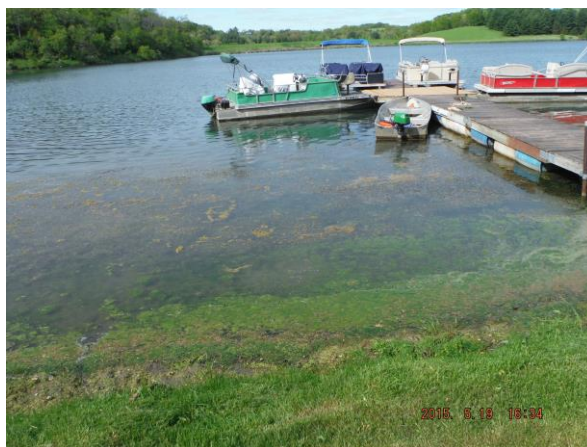
Concession dock, N side
