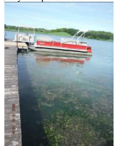
Concession dock, S side
