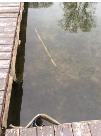
Concession Dock N side
