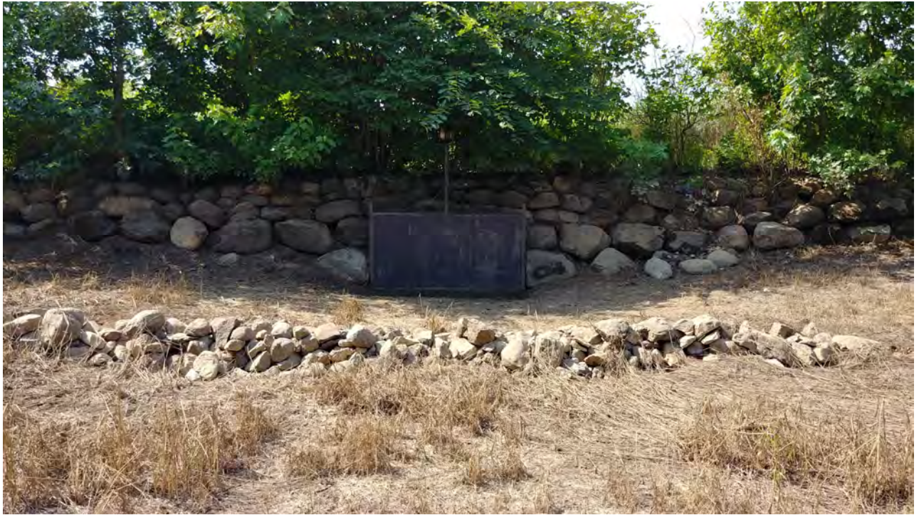
Photograph 5 (7/11/18): Water control structure on north side of access road, looking south.
