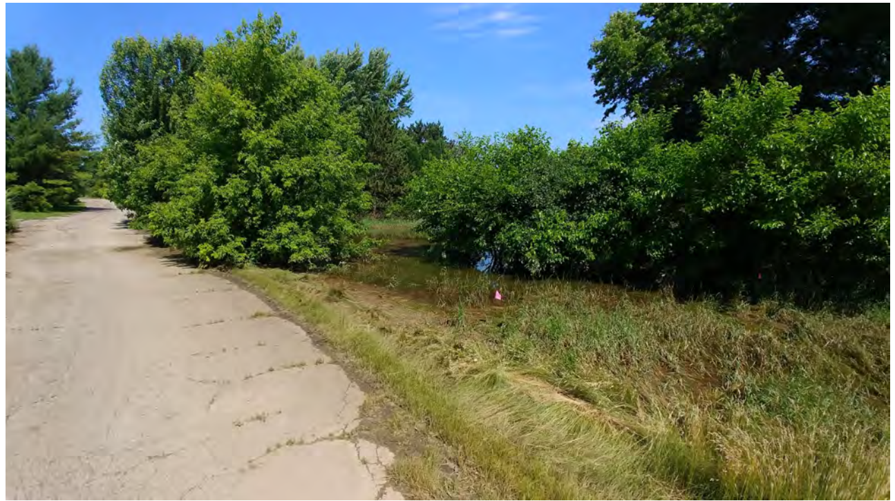
Photograph 3 (6/29/18): Flooded swale, looking west from access road. Bent over vegetation can be seen in the foreground where water flowed over the road.
