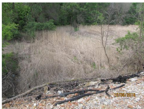
Figure 1: Along railroad tracks east of Danz Avenue
