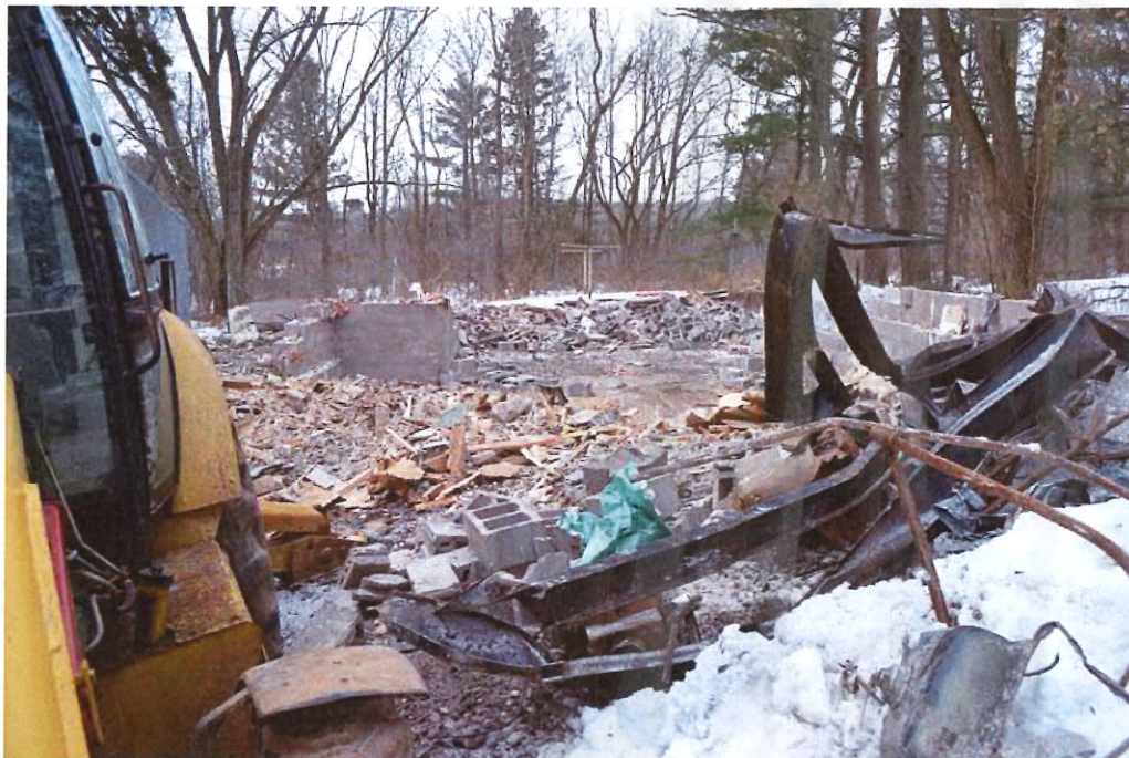
Building Demolition as of January 25, 2017
