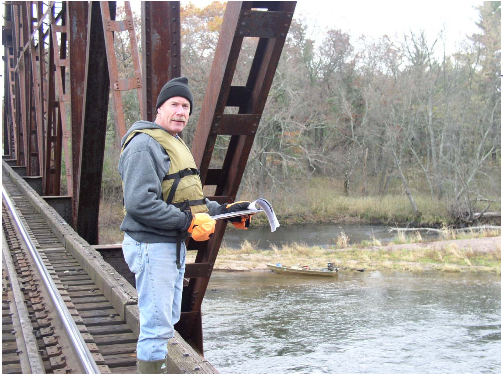
▣ COLFAX RAILROAD BRIDGE
