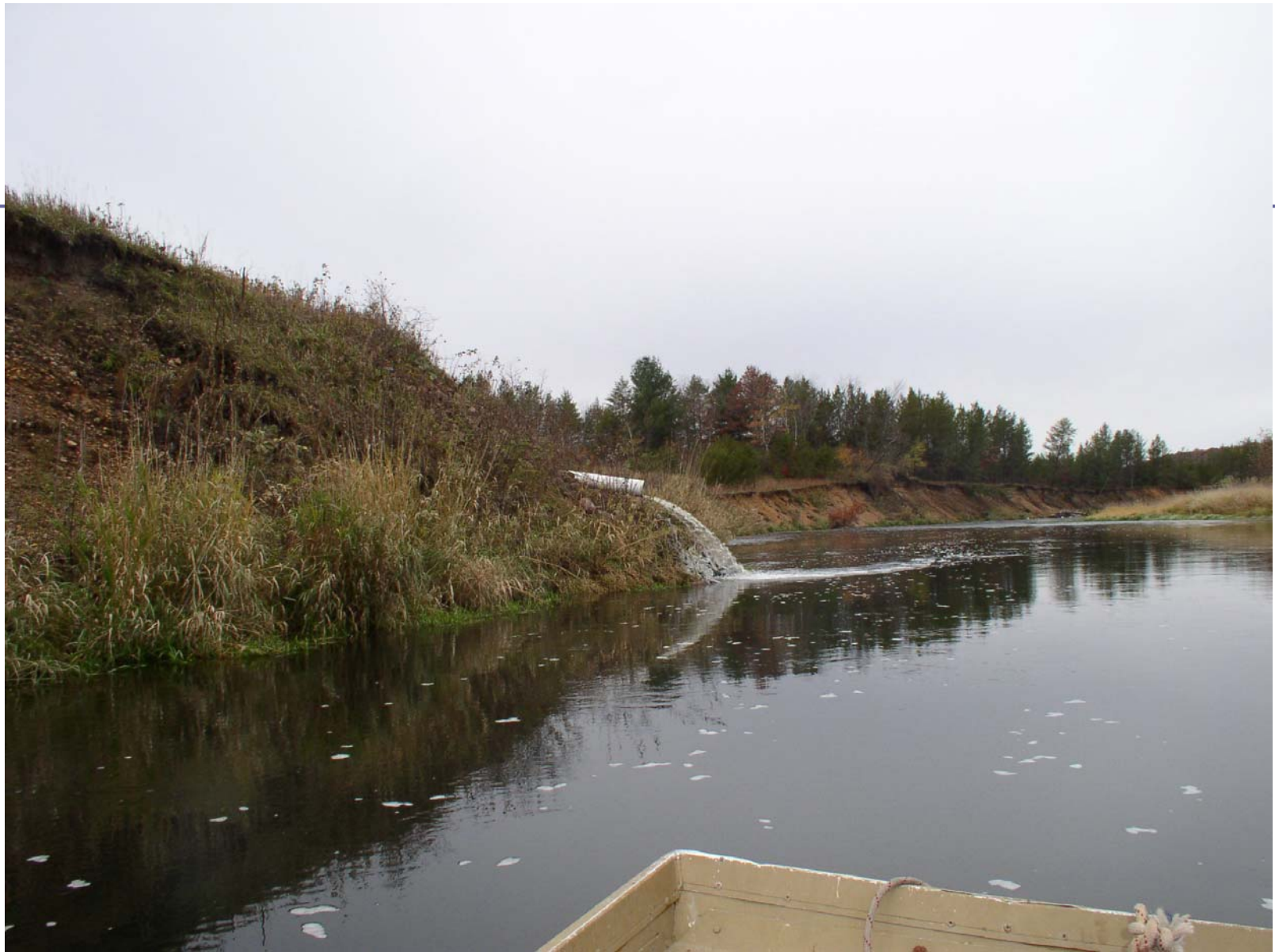
■ COLFAX SEWAGE TREATMENT PLANT DISCHARGE
