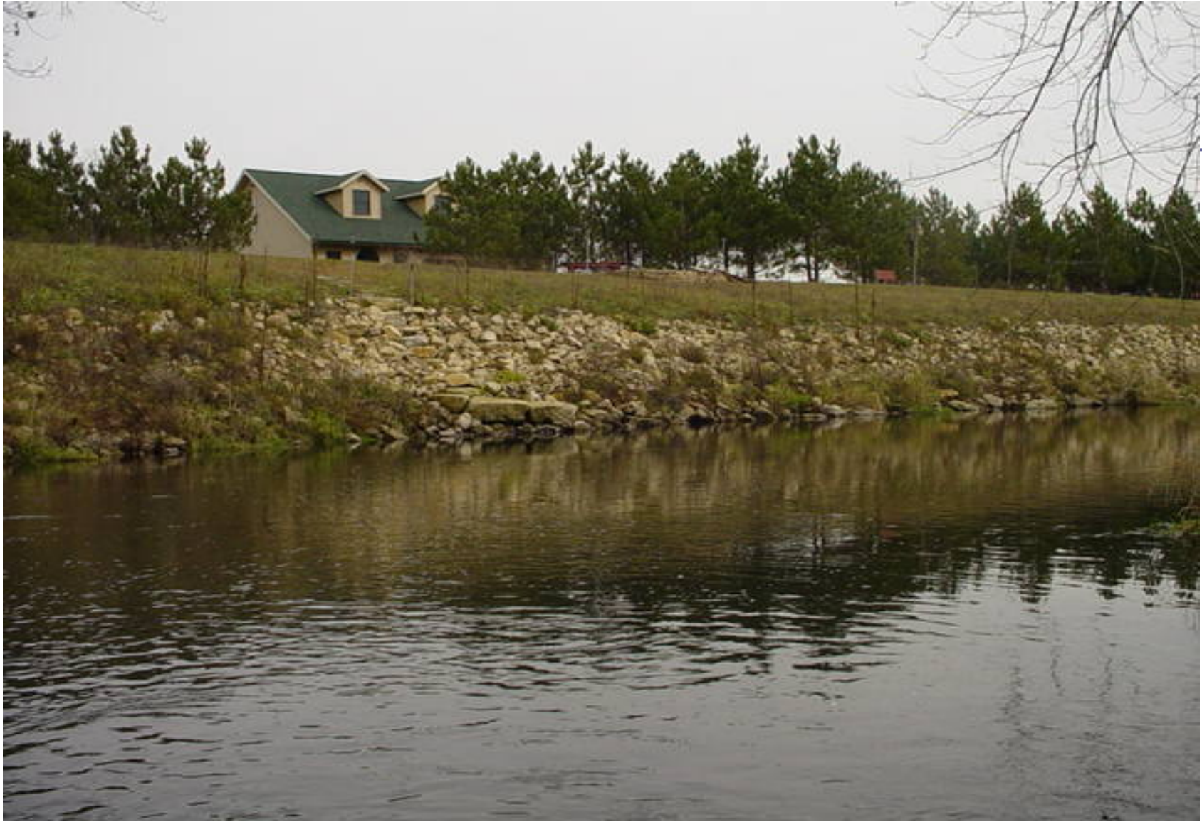
HAY RIVER, RIP RAP INSTALLED IN 2005
