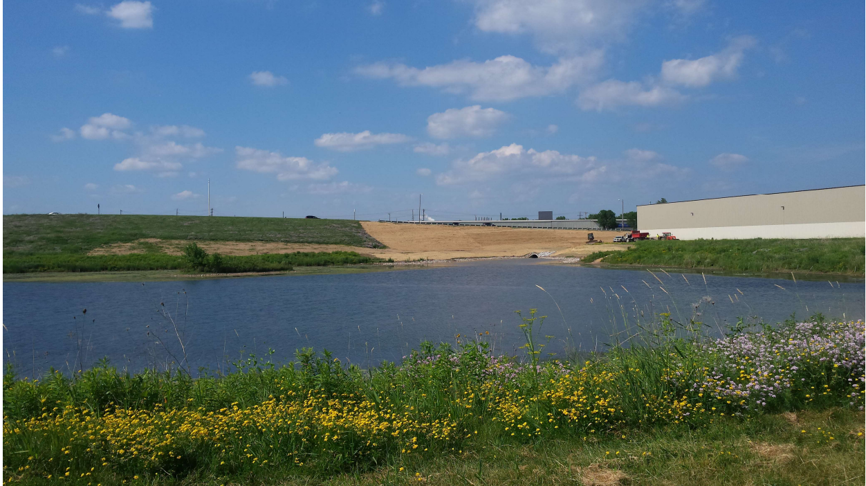
Looking north after erosion mat installation.
