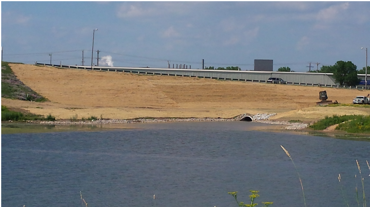
Looking north after erosion mat installation.
