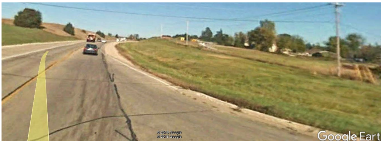
GL207 looking northeast
