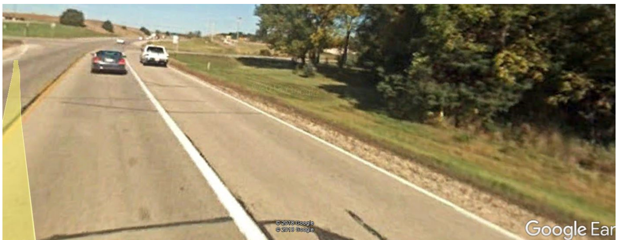
GL209.01 looking northeast
