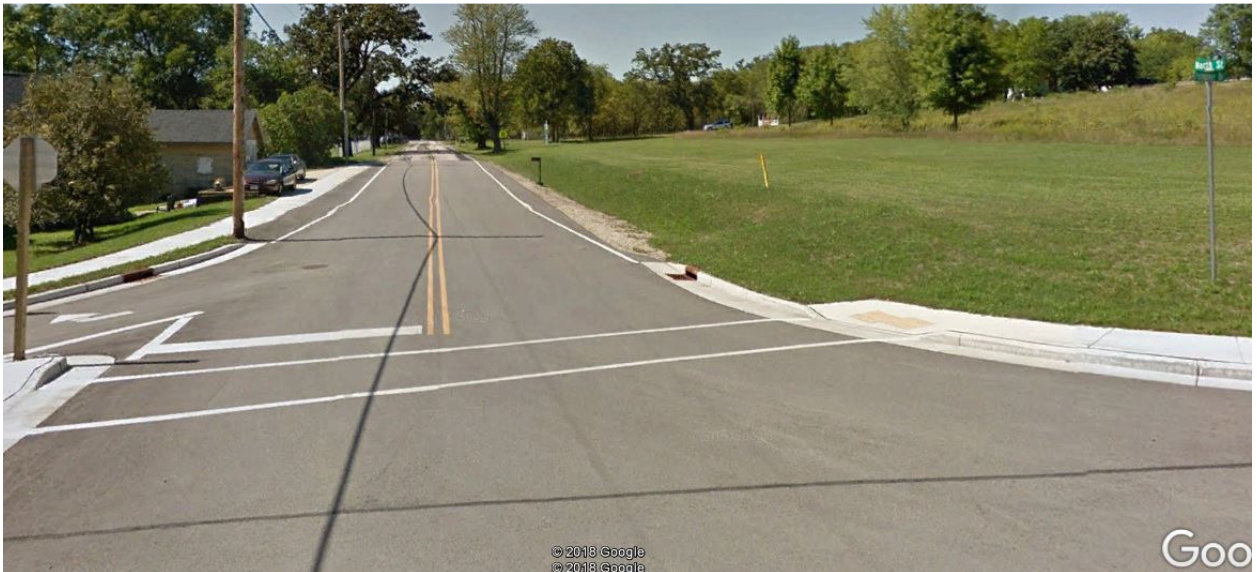
PM200a.02 looking west
