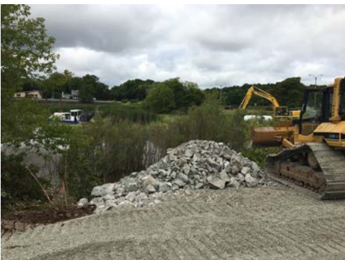
Photo #7 Diversion berm construction
