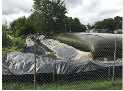
Photo #2 Dewatering area and shoreline protection
