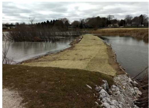
Photo #8 Diversion berm restored
