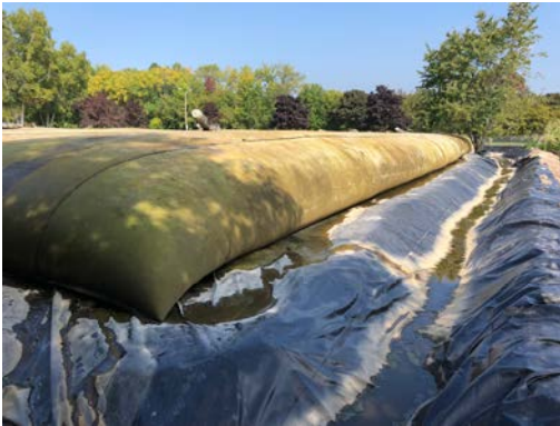
Photo #3 Dewatering area in operation
