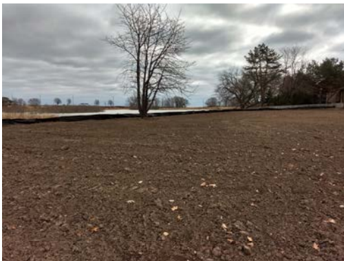
Photo #5 Dewatering area restored with silt fence
