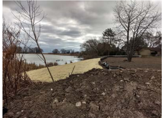
Photo #6 Dewatering area shoreline restored with silt fence
