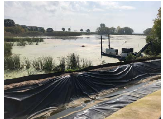
Photo #4 Dredge with dewatering area bank protection
