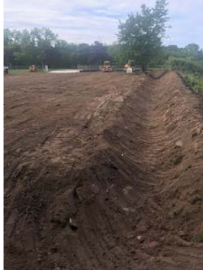
Photo #1 Dewatering area grading
