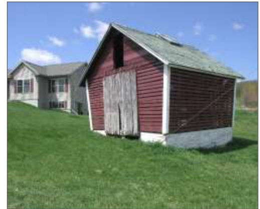
Exhibit 7-1 An example of a rural accessory building
