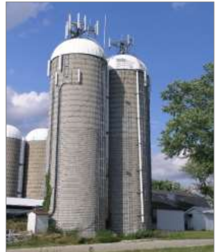
Exhibit 3-2 Two antenna arrays on top of silos
