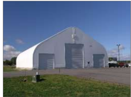
Exhibit 3-5 An example of a polystructure
