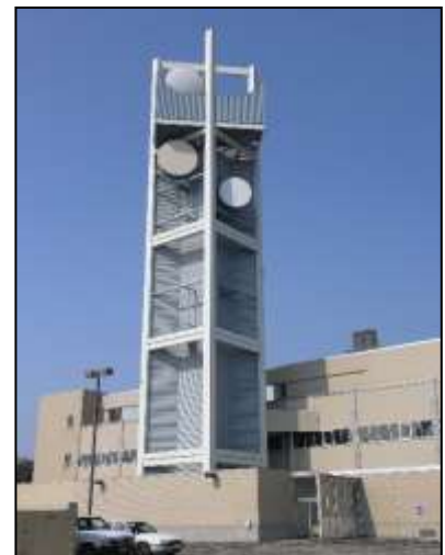
Microwave Tower in Oshkosh
