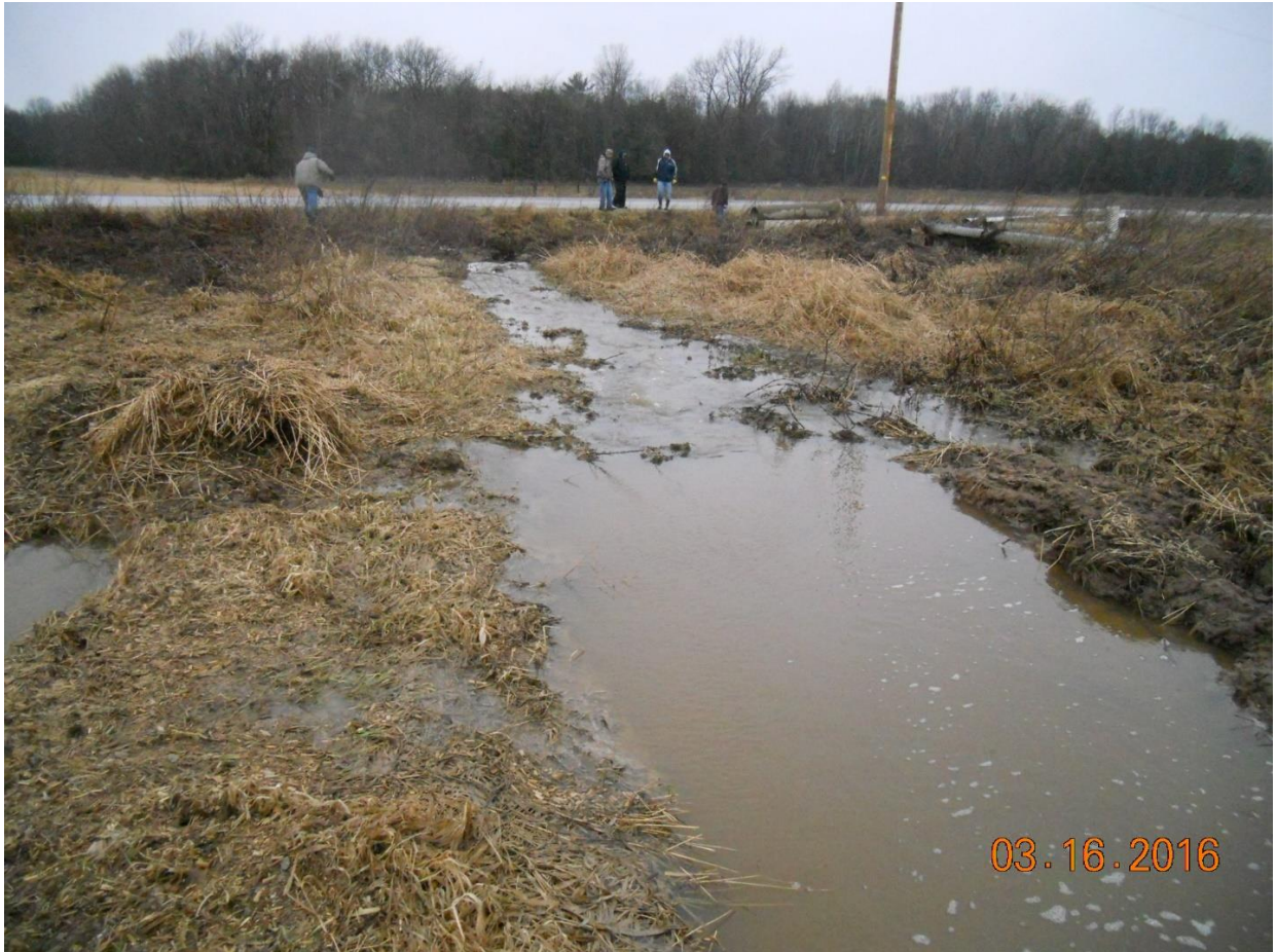
Looking West Runoff entering road ditch
