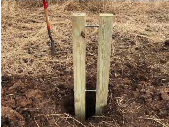
Description: Overview of martin house foundation.
