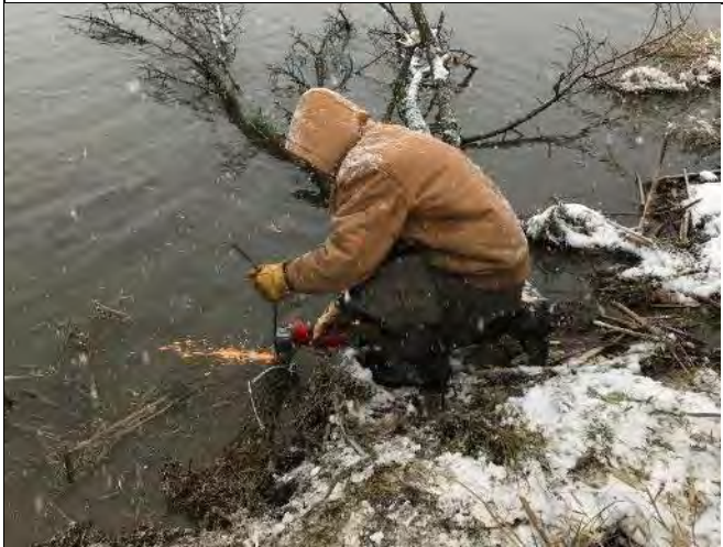
Description: Overview of fish sticks being anchored into the bank.
