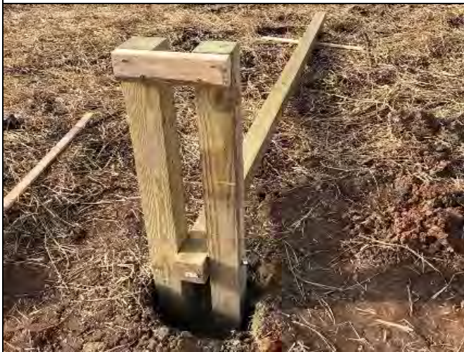
Description: Overview of martin house foundation with mast pole installed.
