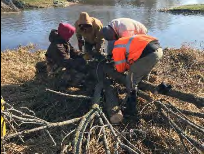
Description: Overview of fish sticks being tied together.
