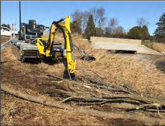
Description: Overview of fish sticks being prepared for installation.
