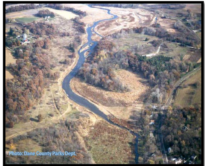
Koshkonong Creek: Newly formed stream channel in what was once an impoundment
