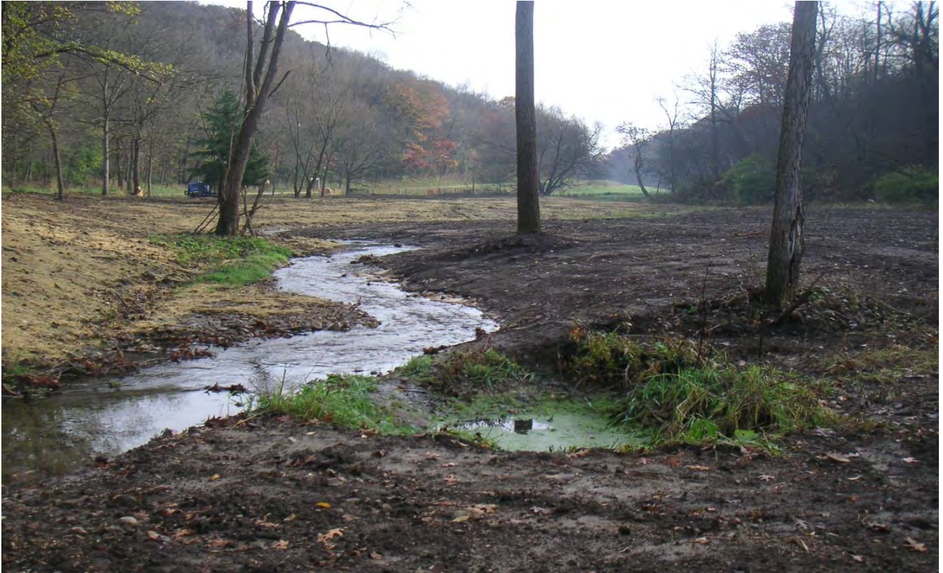
Same site with the berm removed from road to hillside.
