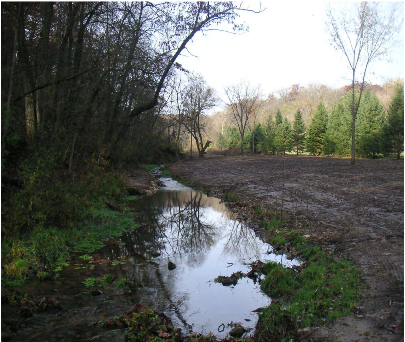
A completed section awaiting seed and mulch.
