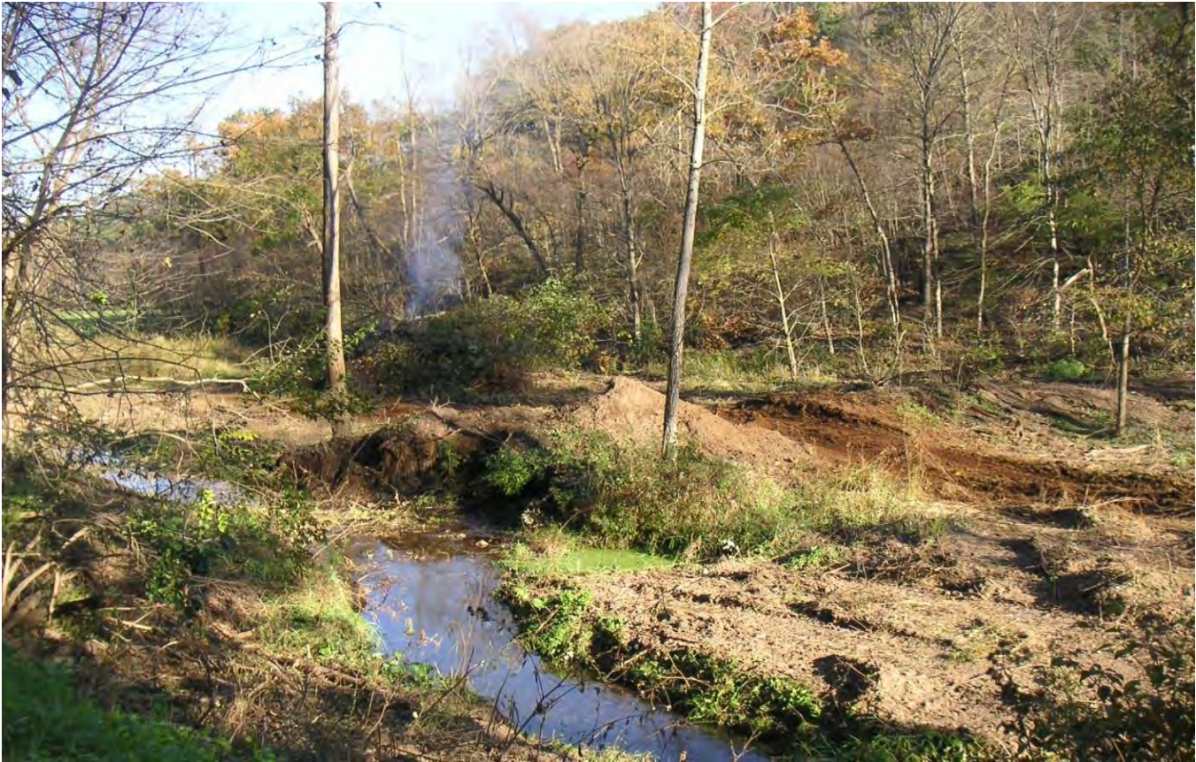
This is the lower earthen berm that was breached when DNR purchased the property.
