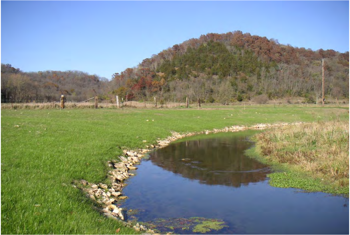
Armored and shaped site from pictures on page 7 with vegetation establishing
