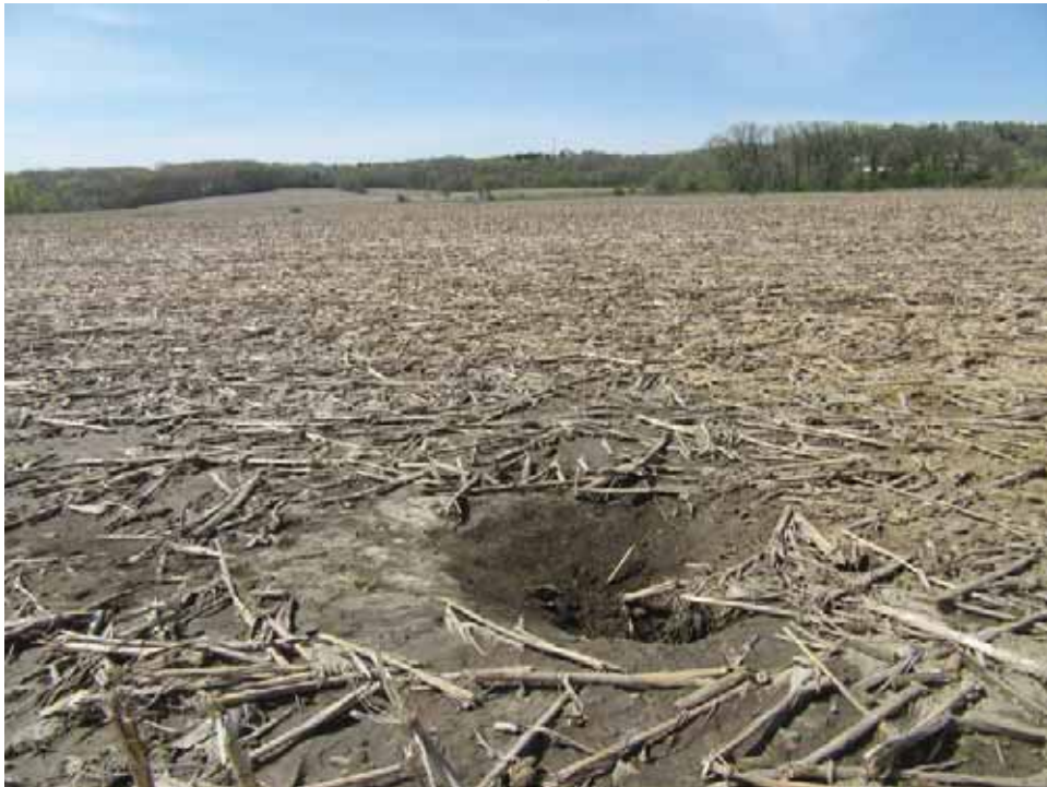
Photo 20. South view, drain tile blowout near sample site 47.
