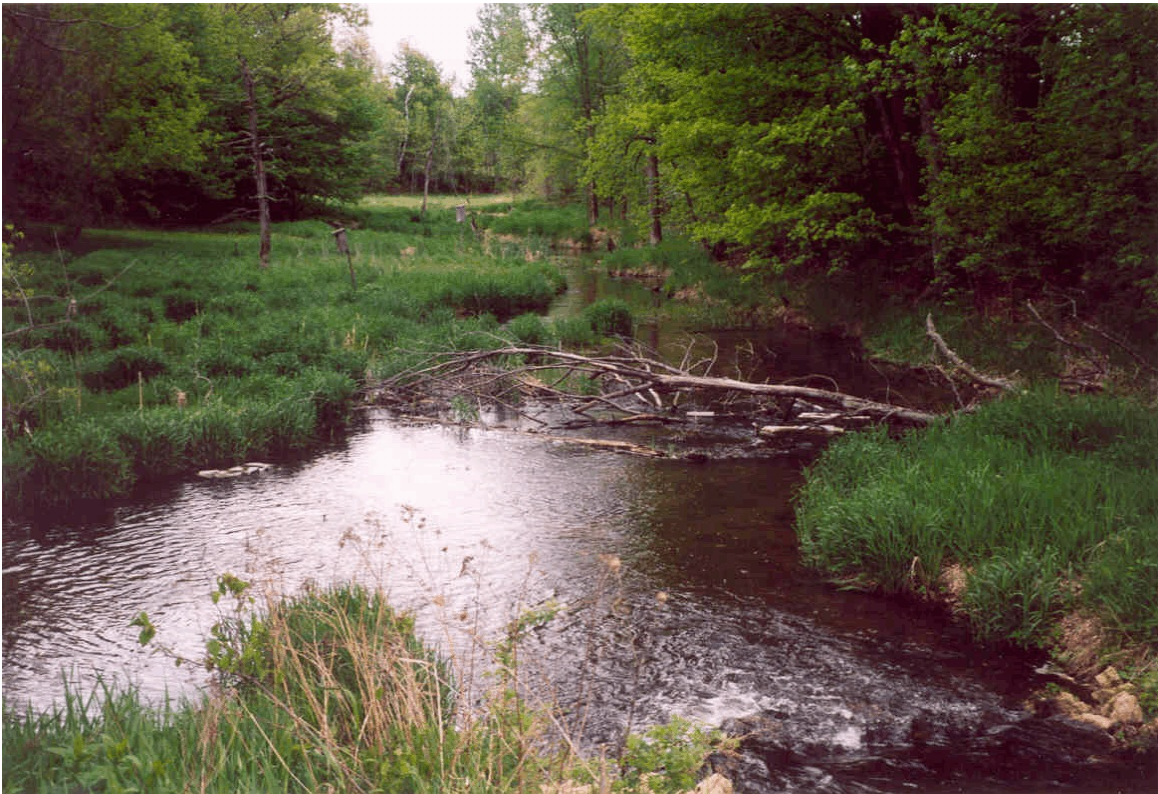
Figure 6. (top) Culverts leaving Upper Turtle Lake that feed the stream that flows into Lower Turtle Lake.
