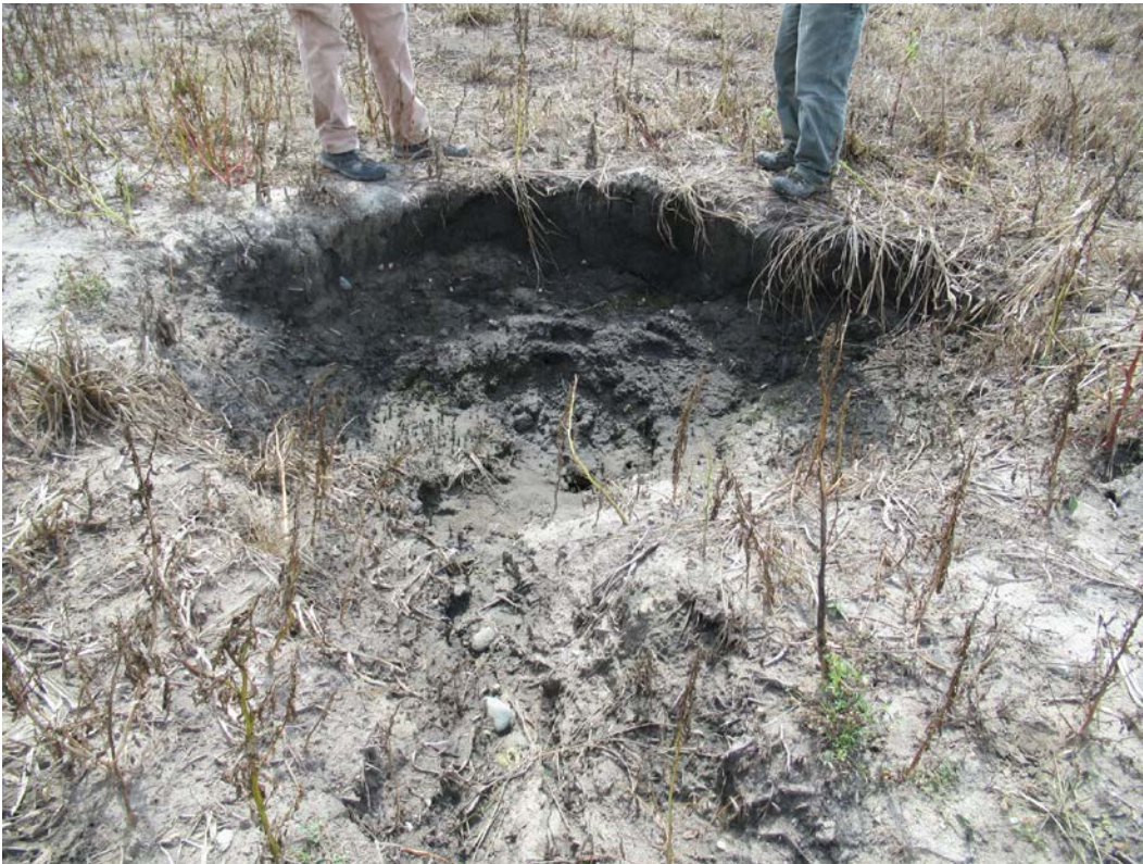
Photo 54. Collapsed drain tile just north of sample site 15.
