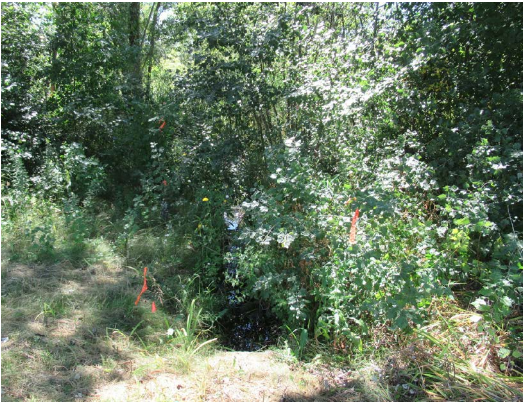
Photo 70. Culvert crossing underneath Durham Drive near sample site 53.
