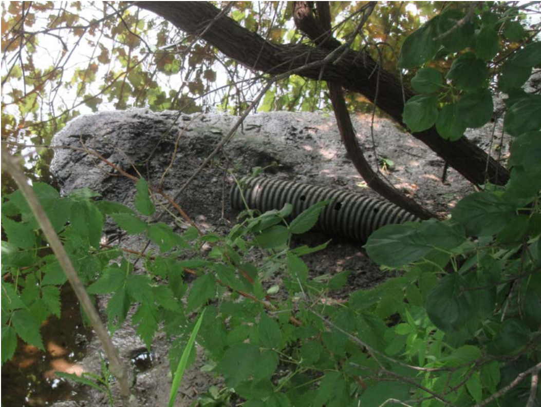
Photo 23. Large drain tile outlet pipe, and associated sediment deposit, just south of sample site 6. The outlet is approximately 7 inches above river level.
